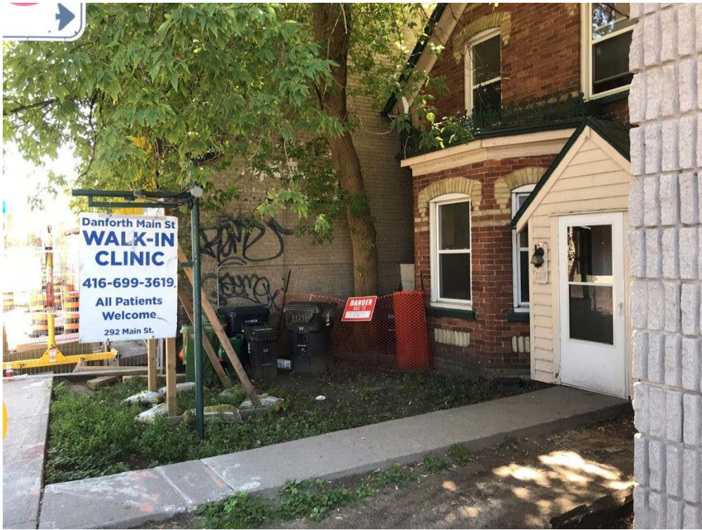
14. View of the subject property looking southwest and showing the setback of the house on the property relative to the later adjacent commercial buildings to the north and south. (HPS, 2018)
