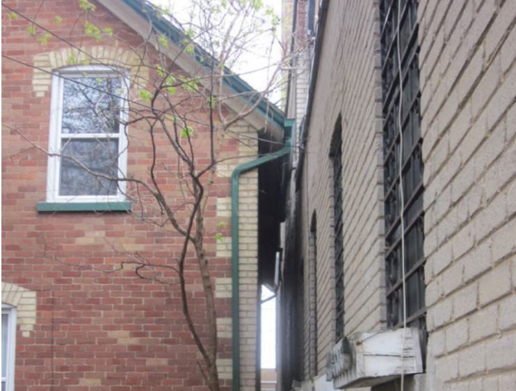
292 Main Street (south west corner)
