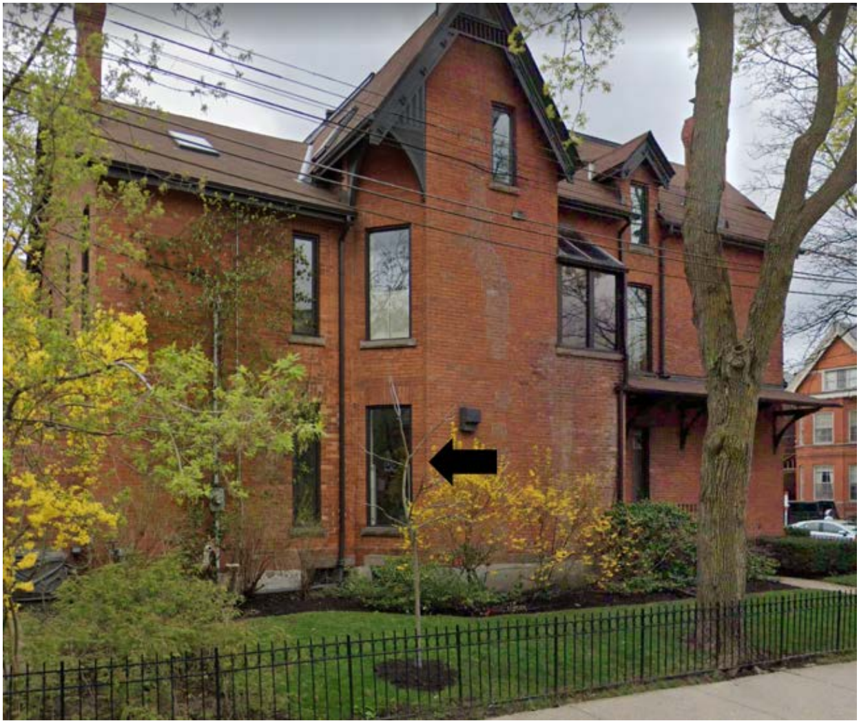
View (facing south) of the existing house at 129 Bedford Road, showing the façade facing Bernard Avenue. The black arrow in this image is indicating the window proposed to be converted to a door
