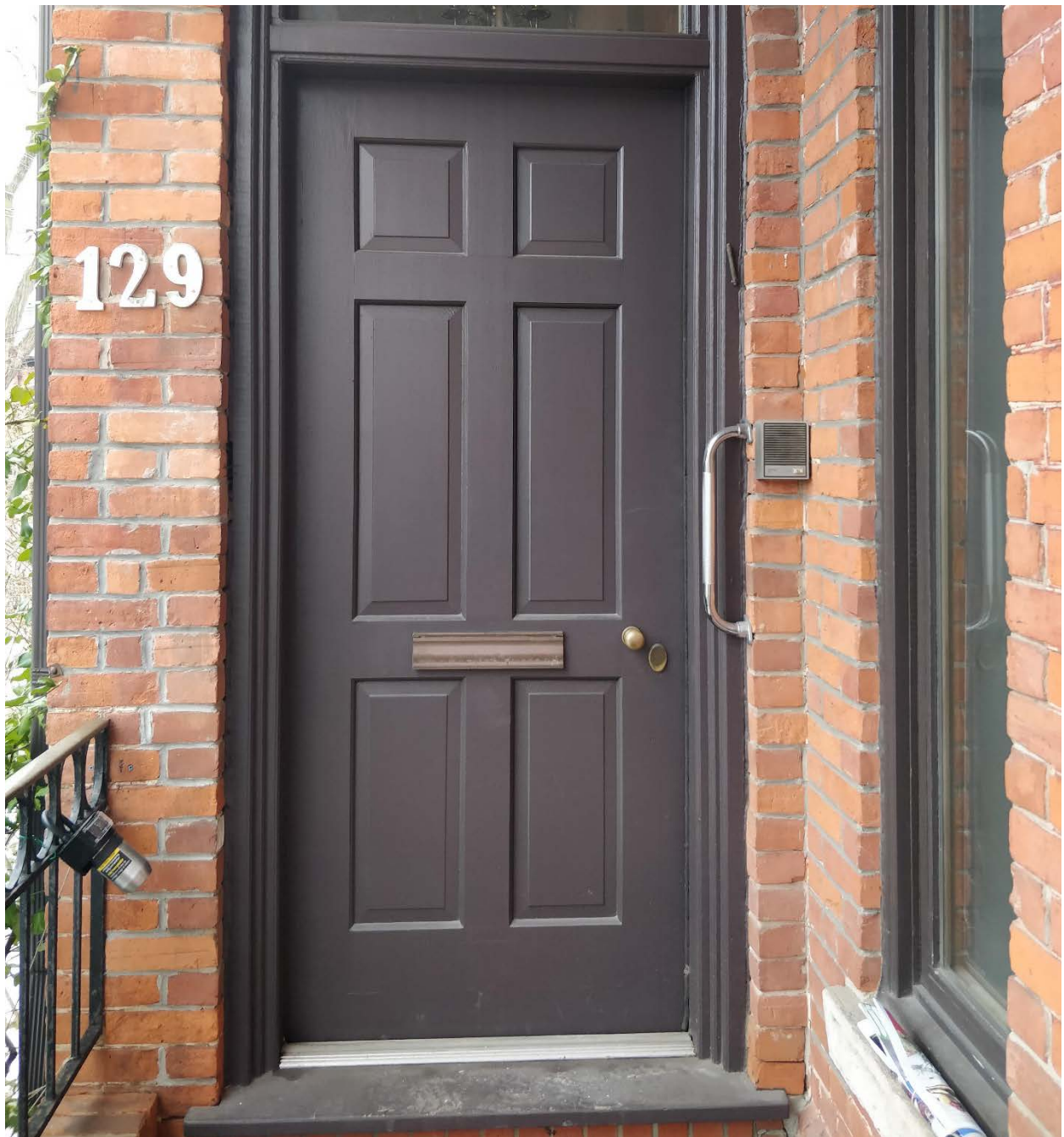
View of existing (non-original) entrance door to 129 Bedford Road that is proposed to be replicated.
