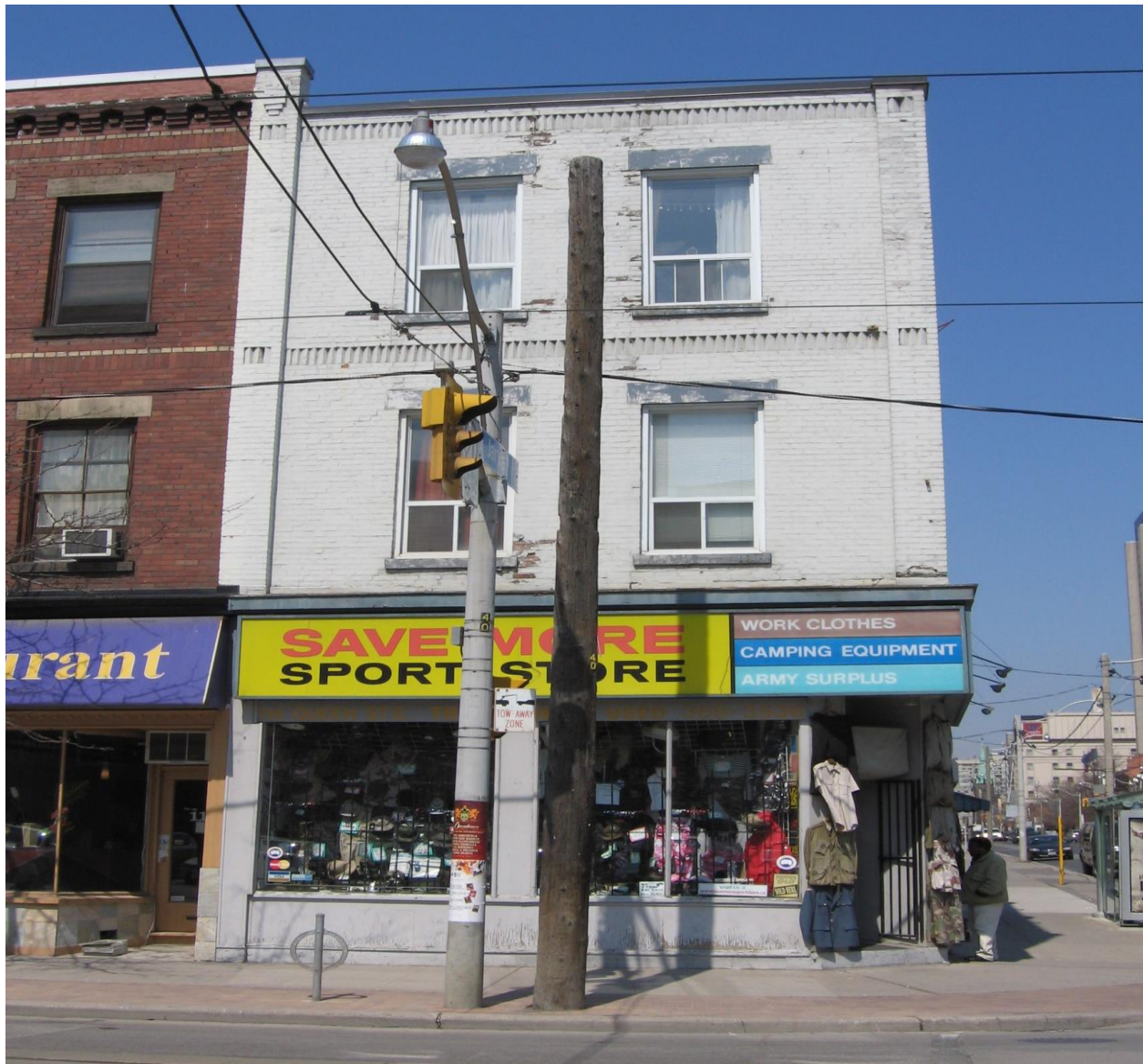
11. Photograph showing the south elevation of 114 Queen Street East with its currently-painted brick cladding and missing parapet, the latter lost sometime before 1973. (HP, 2019)
