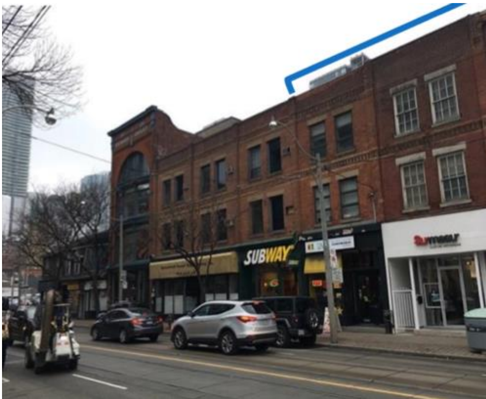
Looking northwest at 106 and 108 Queen Street East (far right and shown with a blue line), with 100-104 Queens Street East that comprise the rest of Mussen Terrace directly left and attached (HP2019).
