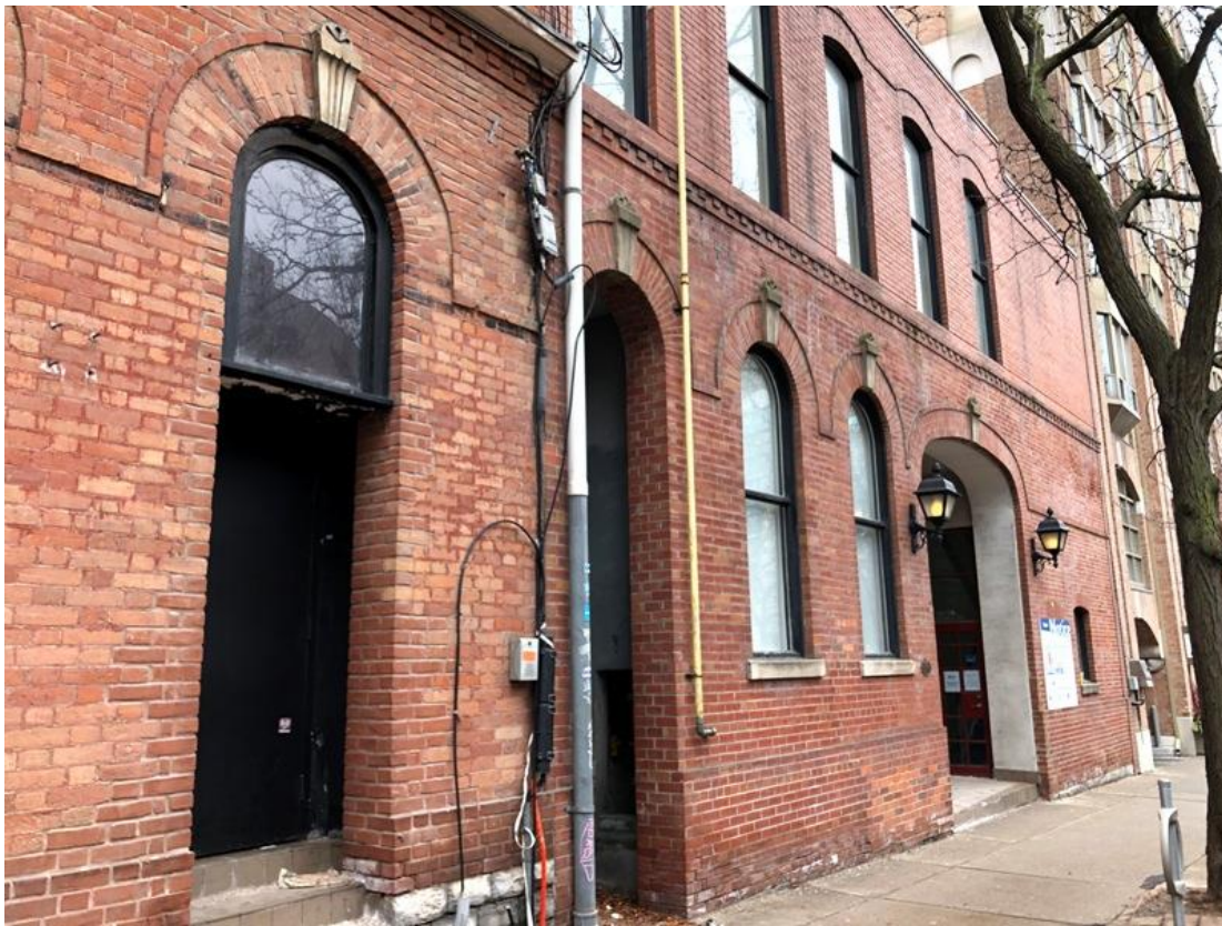
Photograph of the west elevation of the Little York Hotel (left) with its Stables and Coach House (right) (HP, 2020)
