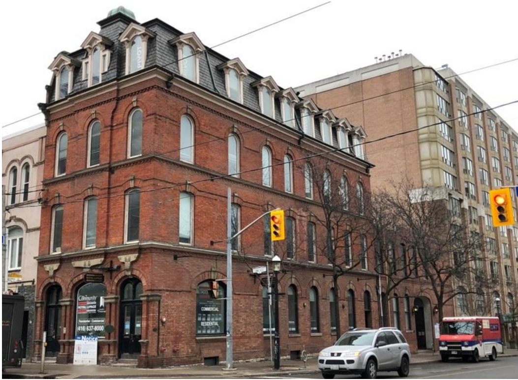
9. Little York Hotel and Stables-Coach House at 187 King Street and 65 George Street (HP, 2020)
