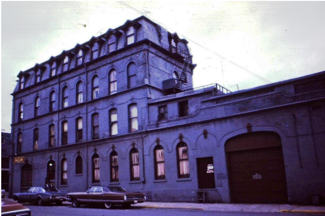
13. 1973 Photograph showing the Little York Hotel complex with the hotel at the left and the stables and coach house at the right. The window adjacent to the stables door was altered to accommodate a shipping entrance c.1945 for a business occupying the ground floor of the hotel. It appears from this photograph that the three windows in the stables building were part of the ground floor space in the hotel. (THB, CTA)
