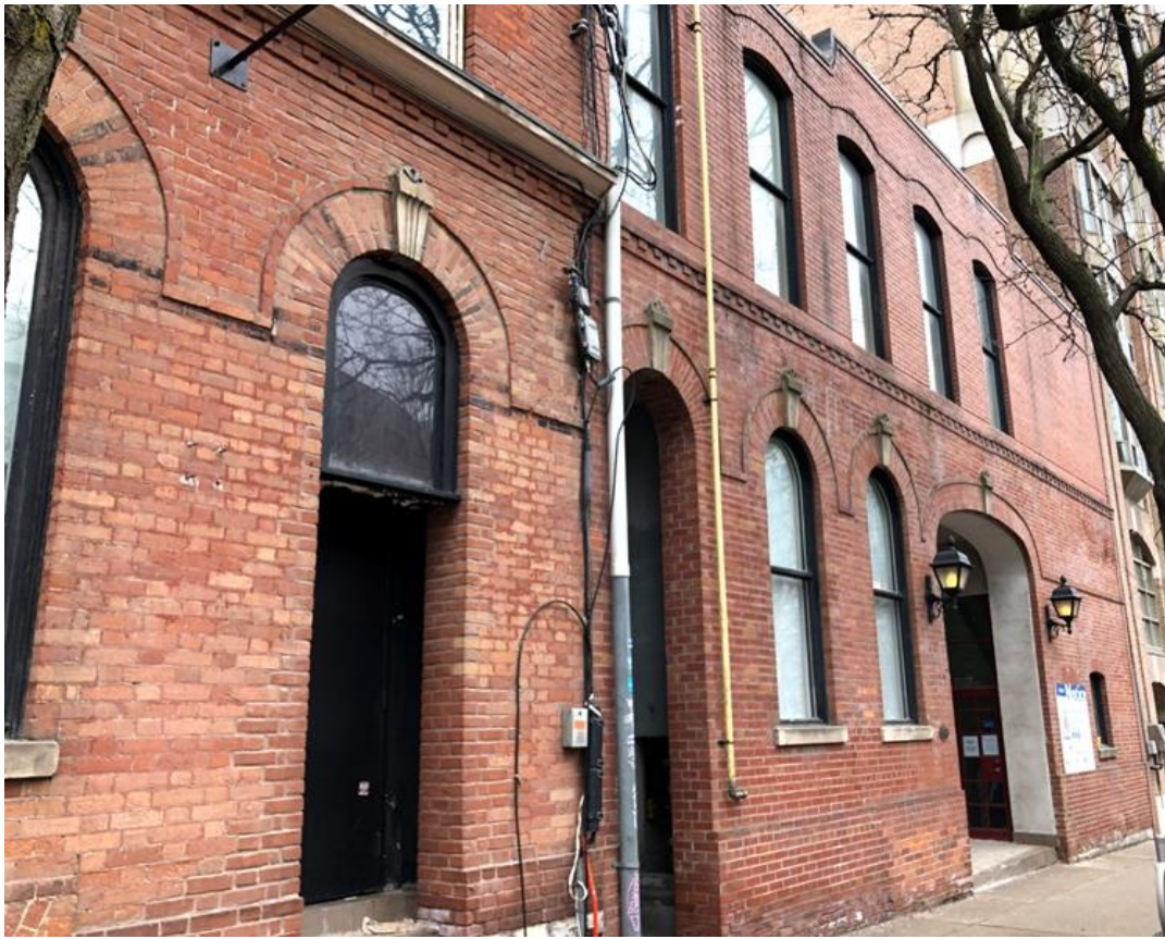
11. West elevation of the Little York Hotel and Stables and Coach House facing George Street (HP, 2020) showing the shared details of the tall round-headed arched windows with stone sills, casts-stone keystones, projecting brick string courses, and dentil course
