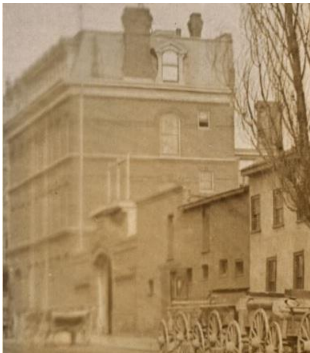
8. Detail of the above photograph, showing the south elevation of the Little York Hotel and the west elevations of the hotel and the carriage way. Note that the current windows to the north of the carriage way entrance do not appear to exist.
