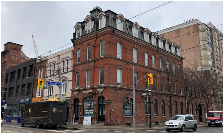
19. Intersection of King and George Streets, south-east corner with the Little York Hotel and Robert Waterhouse's, row of three three-storey commercial buildings, 189-193 King Street East, 1882 (HP, 2020)
