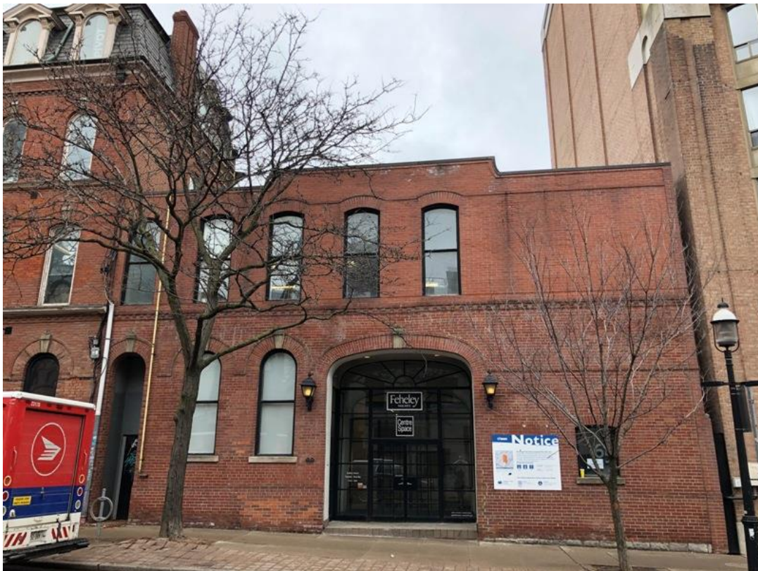
10. Little York Hotel Stables and Coach House adjacent to the Little York Hotel (left)
