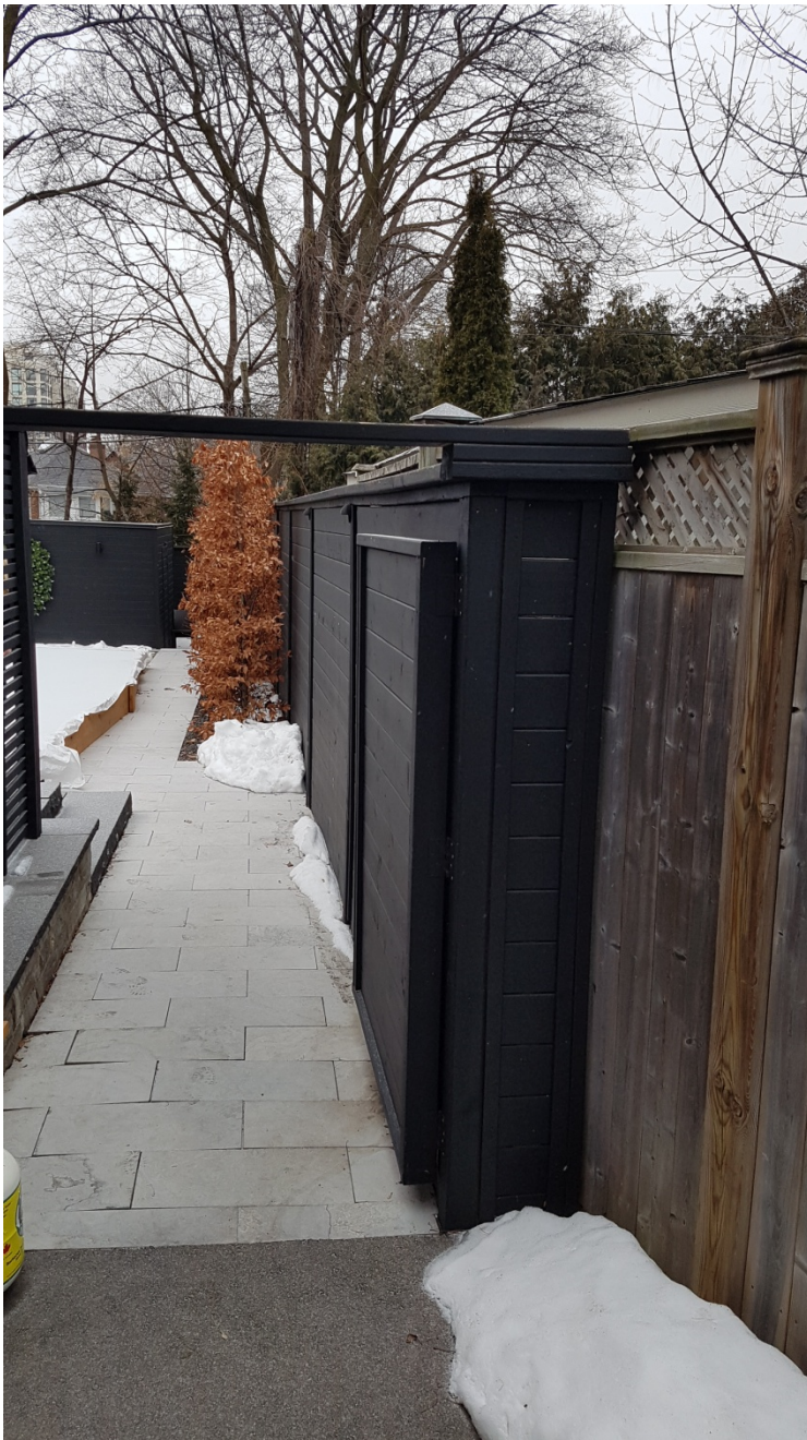
Attachment 2: Existing fence on North side of property (photo taken facing West)
