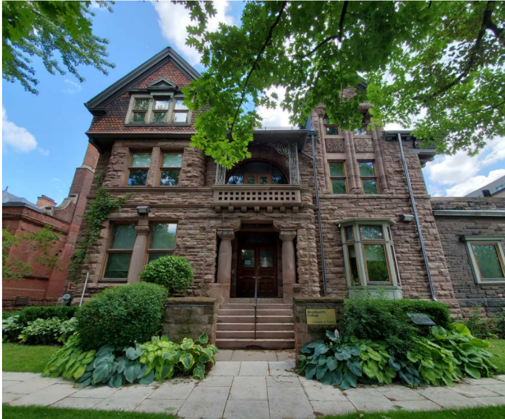
22. Detail of the Alexander McArthur House, principal (west) elevation (Heritage Planning [HP] Photo 2020)
