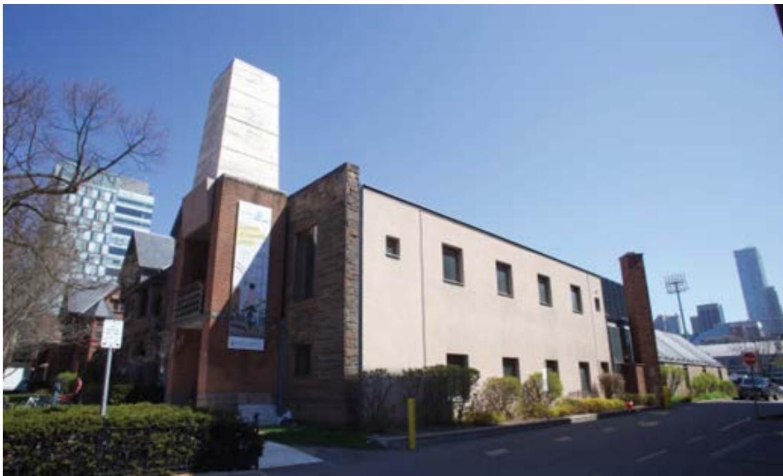
4. 117 St George Street frontage - and south side elevation showing the former officers' quarters
