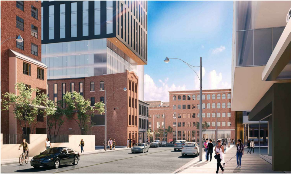
North-west Corner of site (Looking south on Mutual Street) (previous design with lower cantilever)
