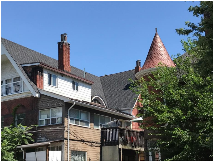
13. Current photograph of 663 Huron Street looking northeast and showing the unique, terracotta colonette clusters supporting the shed dormer roof on the south elevation and the south chimney. (HP, 2020)
