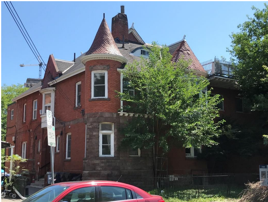
8. Current photograph of 661 Huron Street looking southeast and showing the complicated rooflines of the building, including the main hipped roof, terracotta-tiled conical roofs and centred eyebrow dormer. (HP, 2020)
