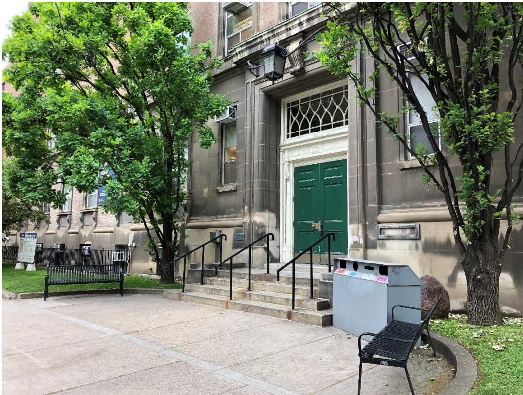
25. Banting Institute, entry forecourt, south elevation facing College Street showing the stone details and cladding of the raised basement and first floor of the central block (HPS, 2019)
