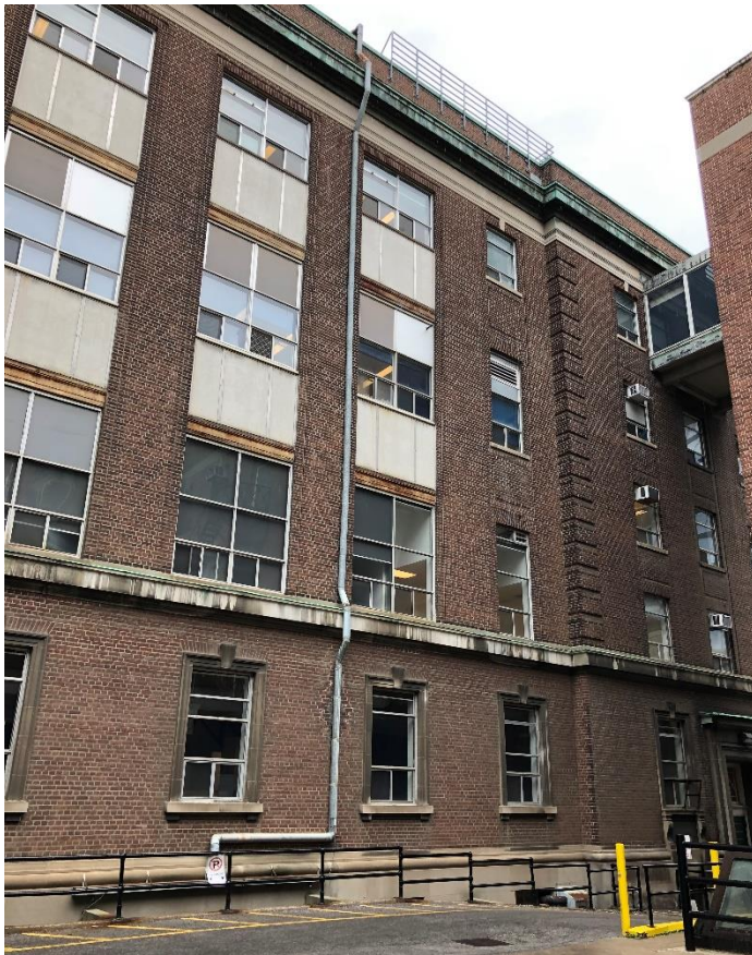
23. Banting Institute (left) showing the side (west) elevation, the side entrance and the bridge to the later Best Institute prior to its demolition. (HPS, 2019)
