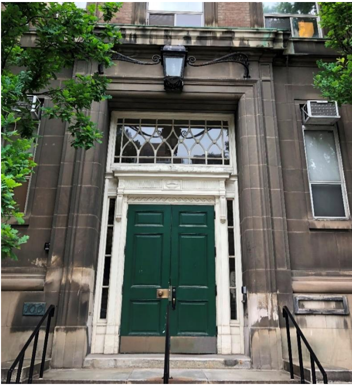
27. Principal entry showing the double panelled doors, wood surround with side lights and tracery in the transom light above, the finely crafted stone of the door frame and cornice with the suspended lantern (HPS, 2019)
