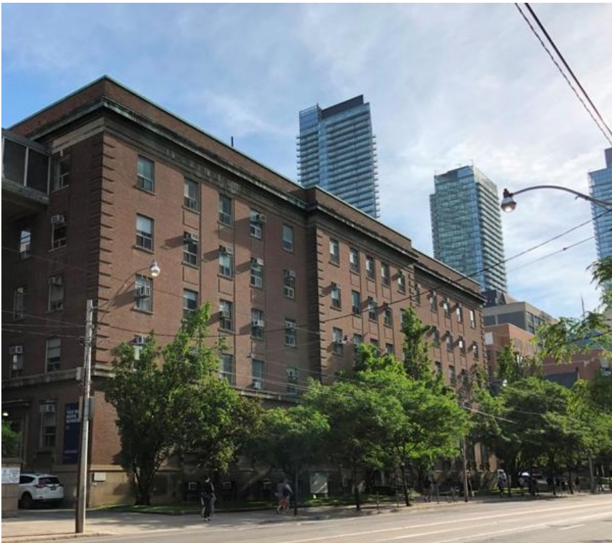
20. Banting Institute, principal (south) elevation facing College Street, viewed from the west. (HPS, 2019)
