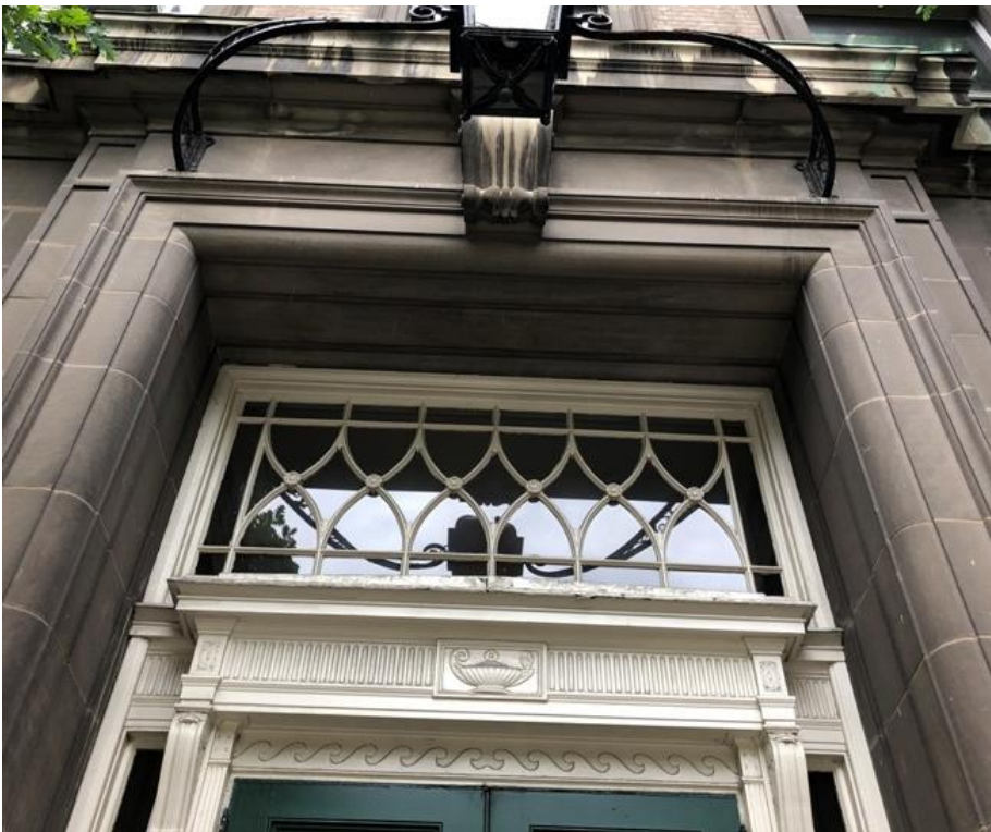
28. Detail of the principal entrance to the Banting Institute showing the various details of the wood door frame and transom including the 'lamp of learning' on the lintel (HPS, 2019)
