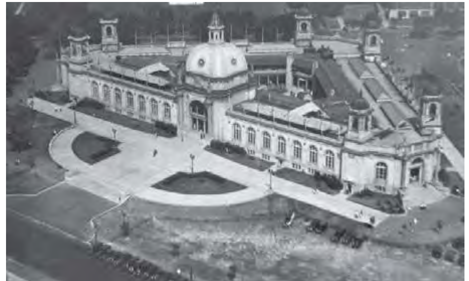
Figure 37. Extract from CHLA - FIGURE 10-8: The monumental scale of the Liberty Grand building is balanced by its generous southwest lawn and plaza (Source: 1929, C.O.T.A., Fonds 1244, Item 2024)
