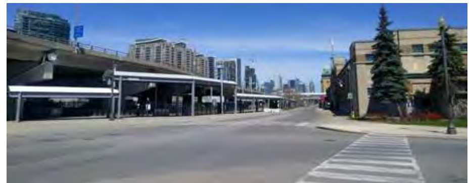
Figure 80. View of Manitoba and Nova Scotia Drives
