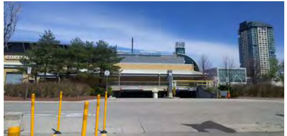
Figure 82. View of underground garage entrance at Exhibition Place
