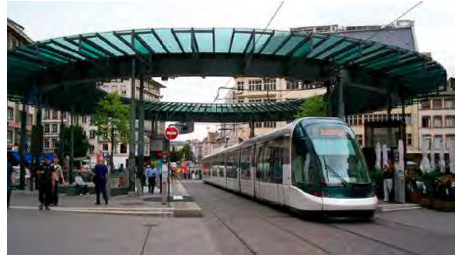
Figure 118. Homme de Fer LRT station, Strasbourg (Source: Eole 99, www.wikipedia.org )
