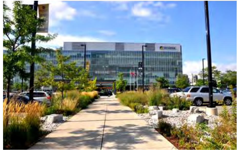
Figure 145. Rain garden in a parking lot
