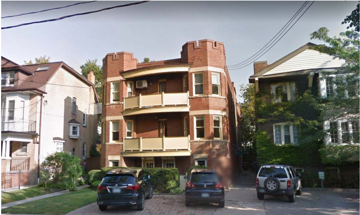
View of the Rosecourt Apartments building at 32 Rowanwood Avenue in 2014 from the south-east.
