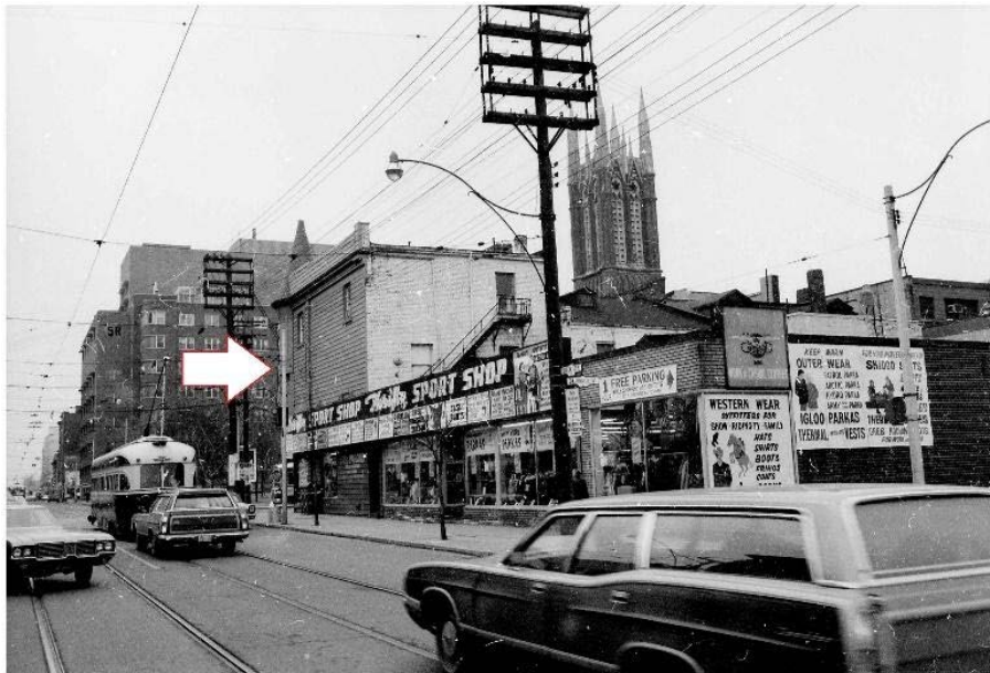
4d. rear of subject properties, 1973, looking west
