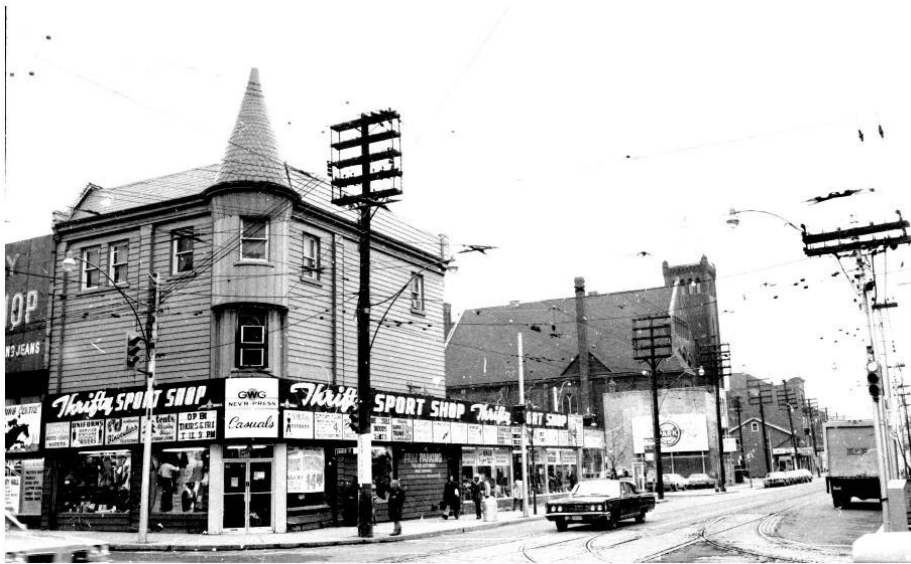
4c. 60 Queen Street East, 1973, looking east
