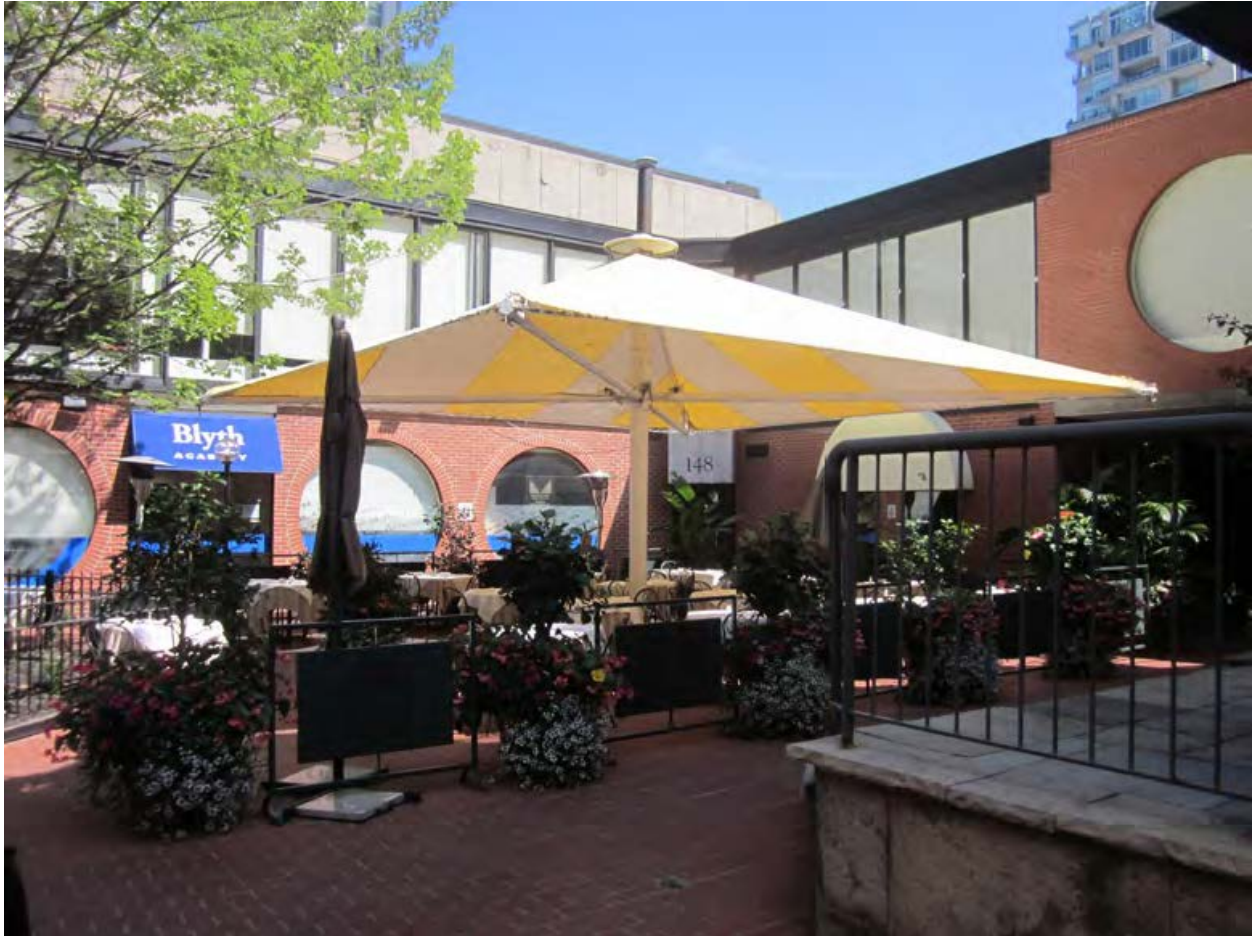
Internal Site - Existing York Square with surrounding 1960s structures
