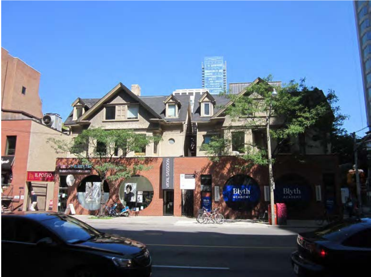
33 Avenue Road - West Facades of Victorian House form buildings. Note 1960s ground level interventions
