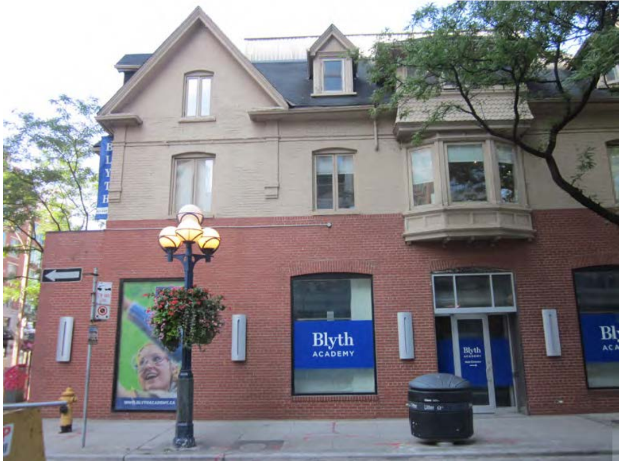
33 Avenue Road - South Facade of Victorian House form building at Yorkville Avenue frontage. Note 1960s ground level interventions
