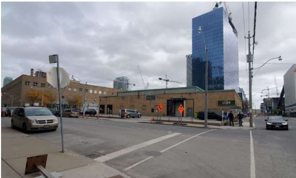
19. Detail of the original garage south of the Warehouse that has been remodelled into a retail store (Heritage Planning, 2020)
