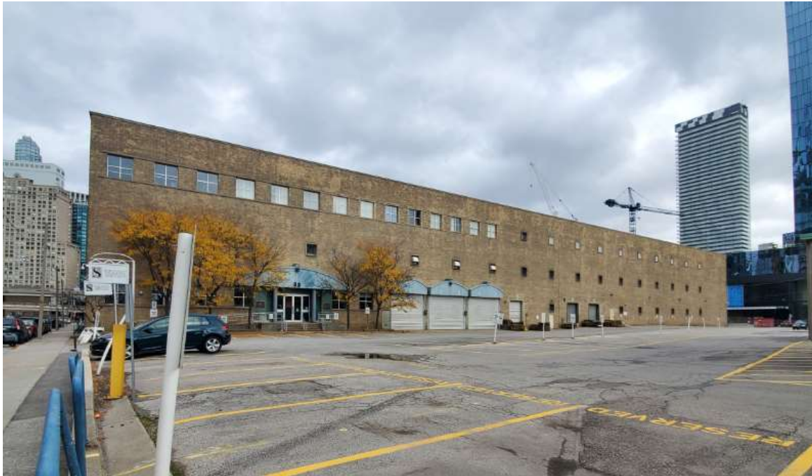
18. Detail of the south elevation of the Warehouse fronting Queens Quay East (Heritage Planning, 2020)
