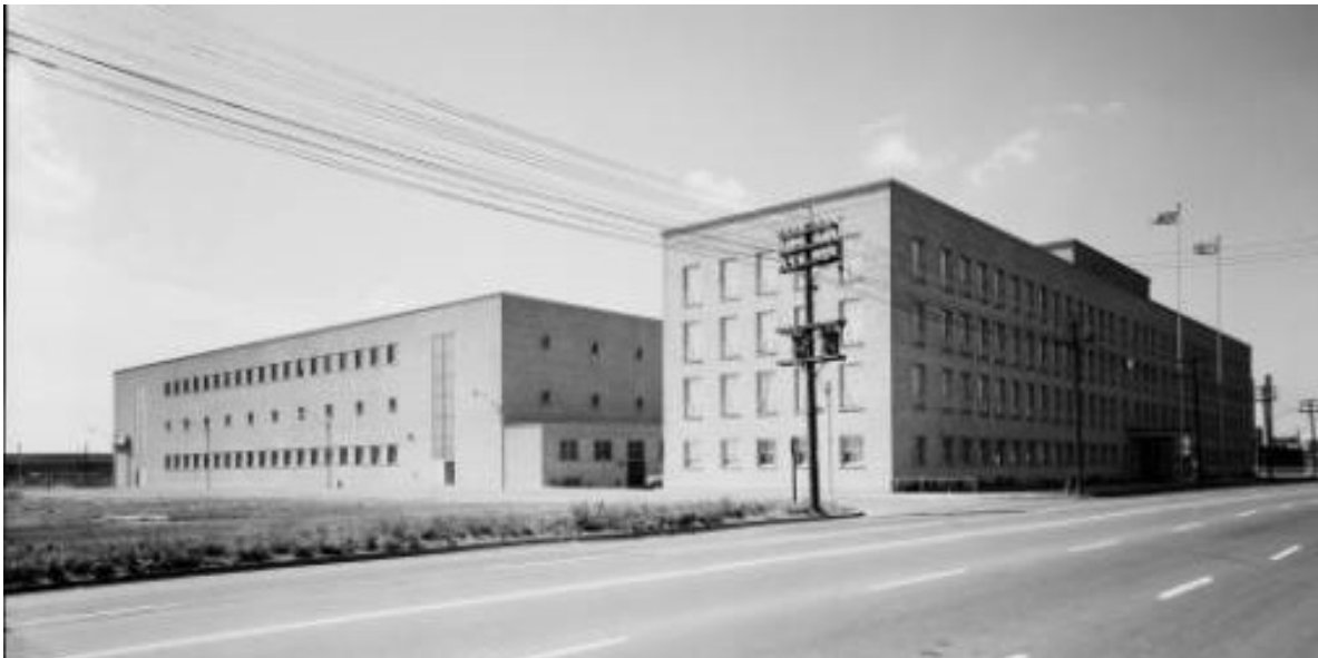
Archival photograph showing the east (side) elevations of the LCBO Office Building (right) and Warehouse (left) (1955) (Panda Associates, Canadian Architectural Archives)
