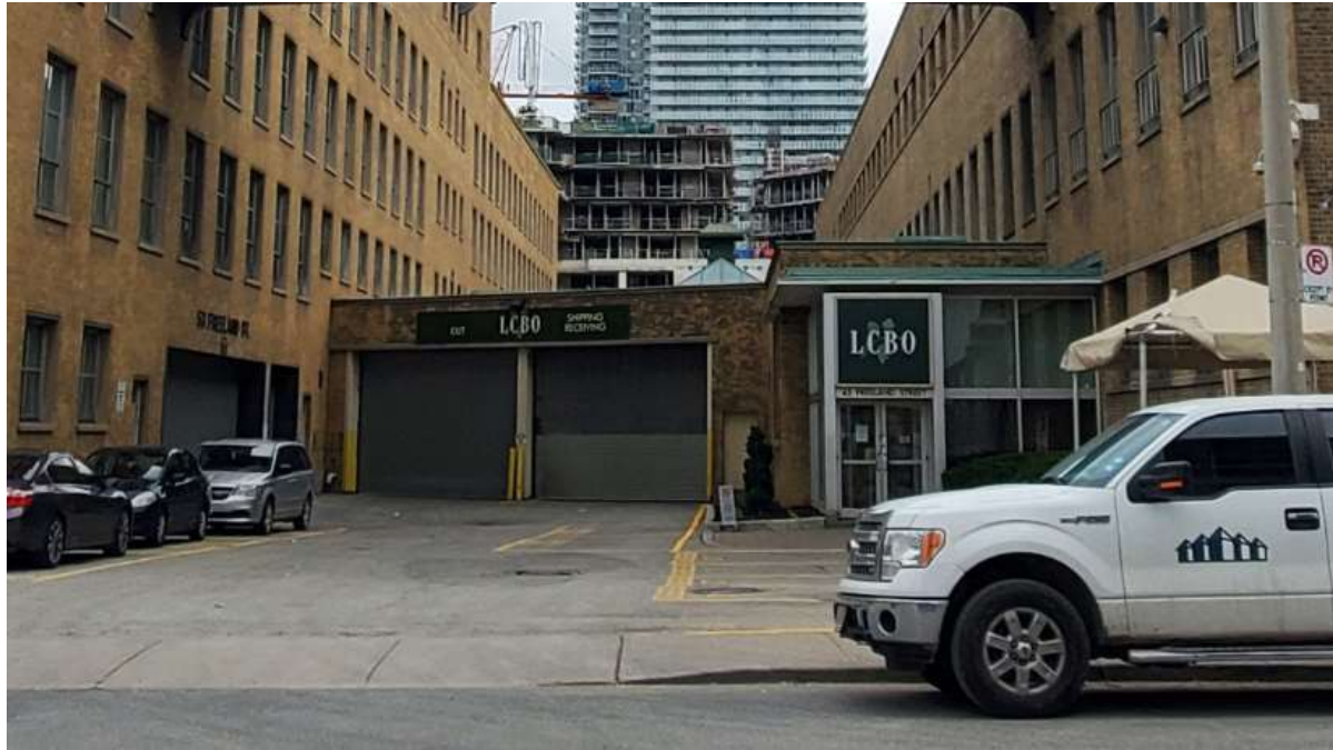
16. Detail of the side (west) entrance to the Warehouse and the rolling garages in the one-storey connecting building (Heritage Planning, 2020)
