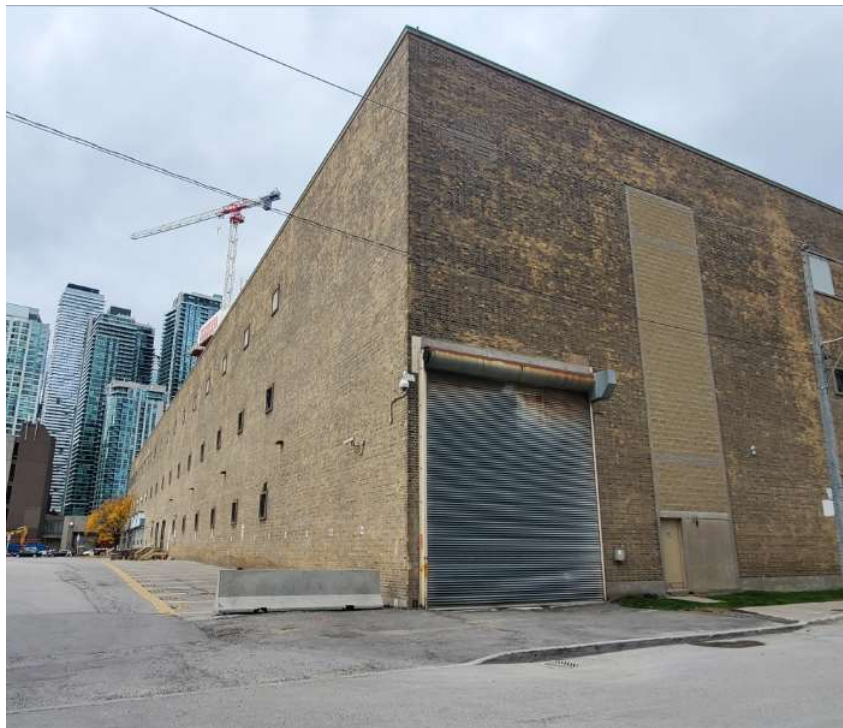
17. Detail of the garage at the south end of the side (east) elevation of the Warehouse (Heritage Planning, 2020)
