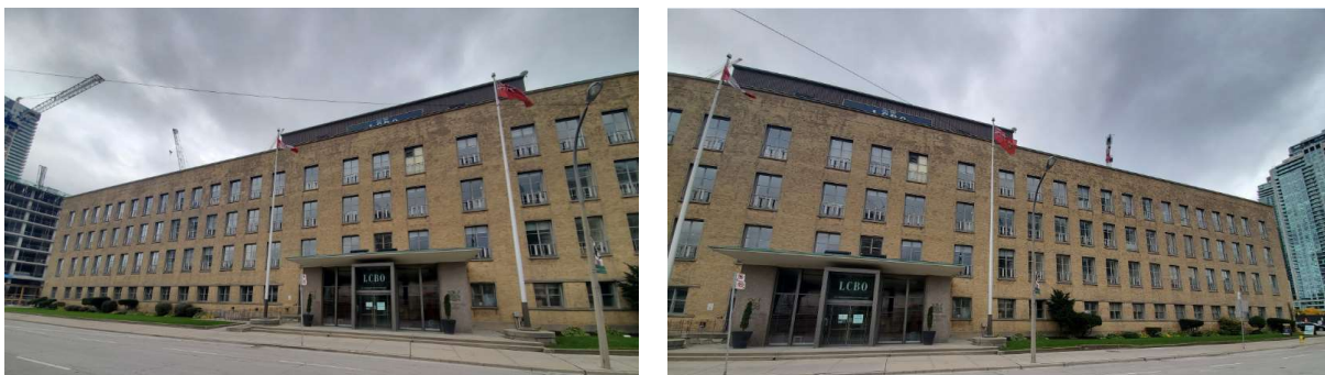
11a and 11b. Details of the principal (north) elevation of the LCBO Office Building (Heritage Planning, 2020)
