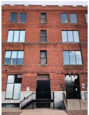
30. North Elevation, 135 Liberty Street showing the details and the original loading dock opening with transom light and original sash windows above, concrete base, cast cement sills, cement belt courses. (HP, 2020)
