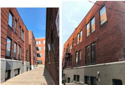
43. View (left) of the south elevations of 47 and 49 Fraser Avenue along a passageway terminated by 53 Fraser Avenue. Note the bilateral symmetry of the projecting outer bays, the pattern of striated brick work creating piers between windows with decorative panels beneath the windows on 47 Fraser Avenue (HP, 2020) 44. View (right) of the rear elevation of 47 Fraser Avenue (HP, 2020)
