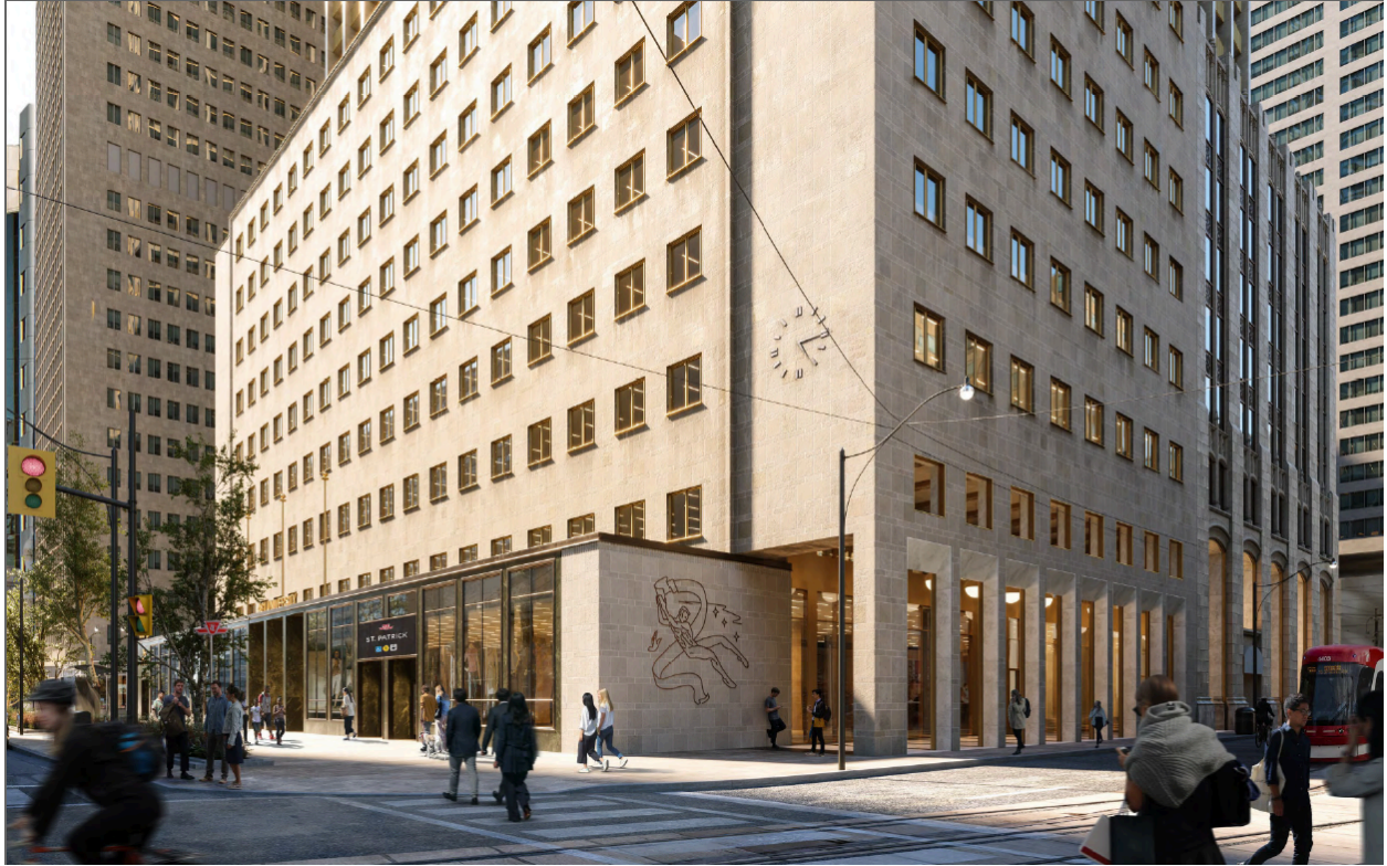
Figure 5 - VIEW FROM SOUTHWEST SHOWING ART SITE CONTEXT
