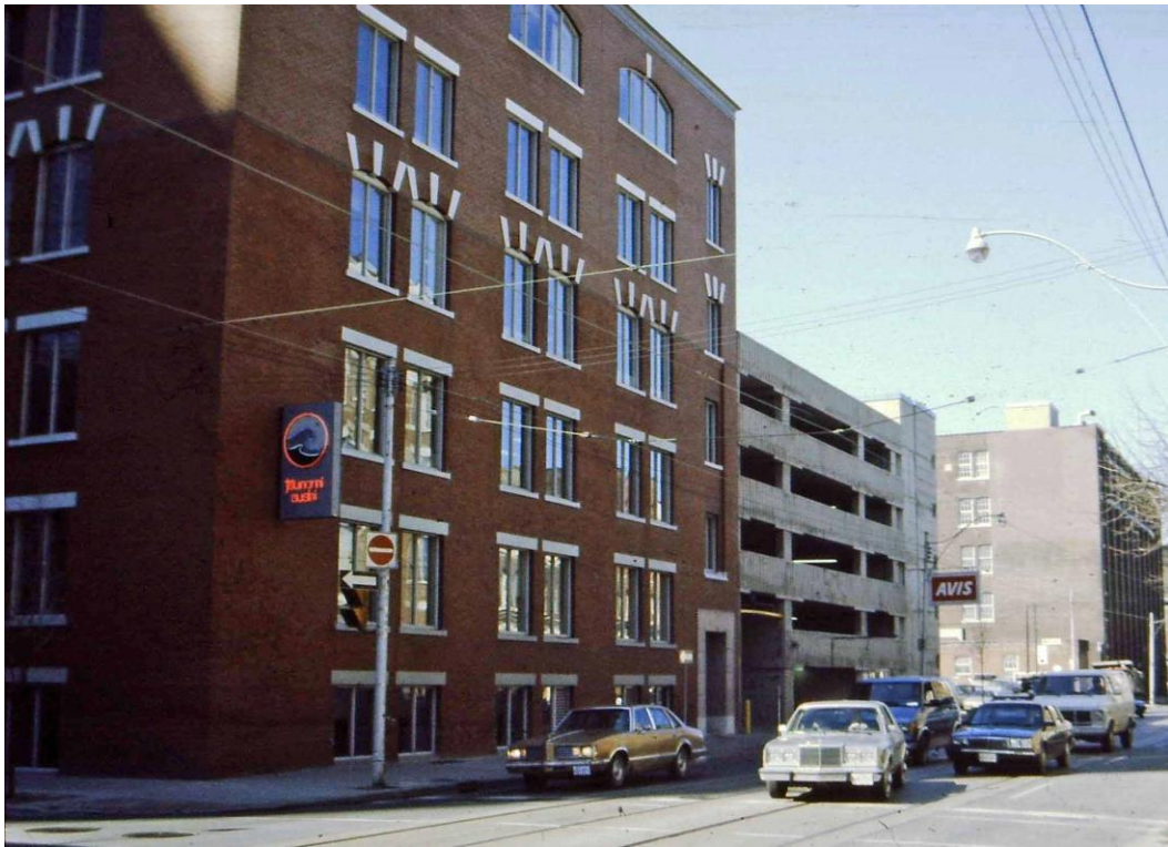
14. Archival Photograph, 100 Simcoe Street, 1988: showing the north elevation of the complex on Adelaide Street West after the addition of the complementary fifth storey (Toronto Historical Board).
