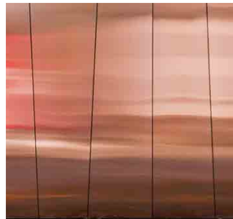
SEALED COPPER CLADDING
