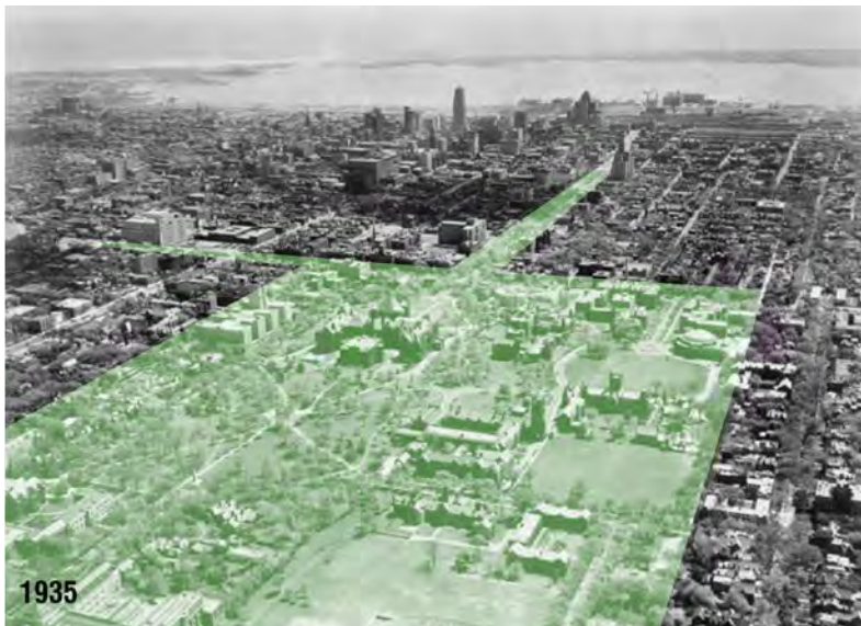
5. Diagram highlighting area of park lots that composed the original Queen's Park and U of T site prior to creation of Queen's Park Crescent West; image ca. 1935. (Source: Toronto Archives, annotations added by ERA Architects Inc.)
