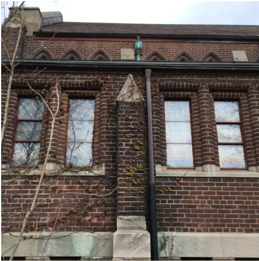
South elevation showing vine growth and damage; and missing windows - typical (ERA, 2020).
