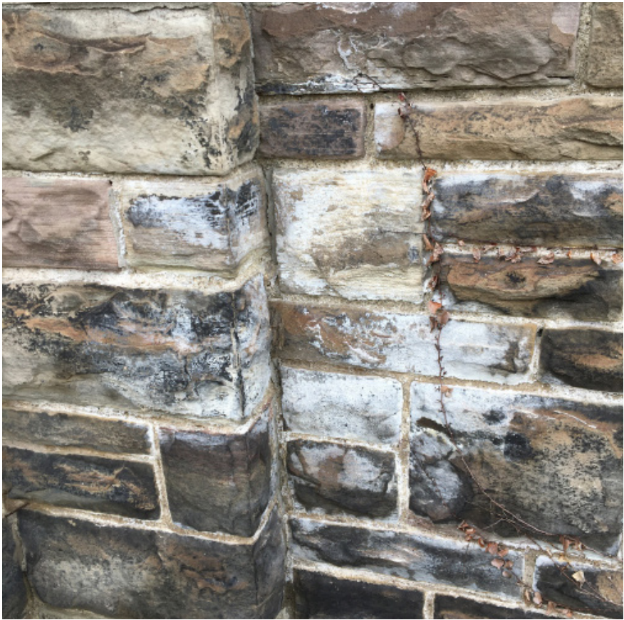
Efflorescence on ashlar base - typical (ERA, 2020).
