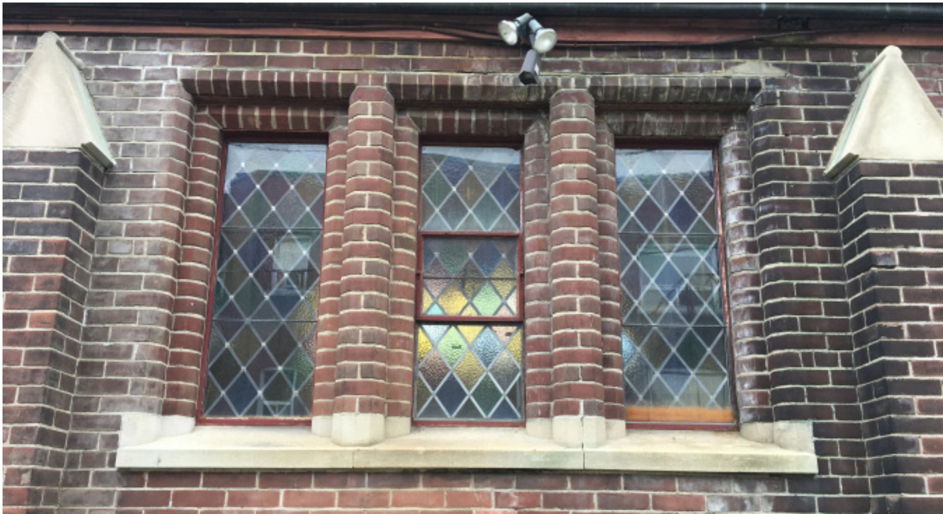
North elevation showing spalling brick, environmental staining, efflorescence, face brick erosion from clinging vines and miscellaneous ferrous metal penetrations/services on the exterior of the building - typical (ERA, 2020)
