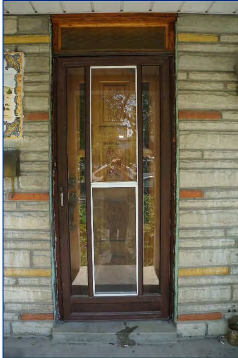
Figure 33: View north of 40 Mitchell Avenue main entrance door
