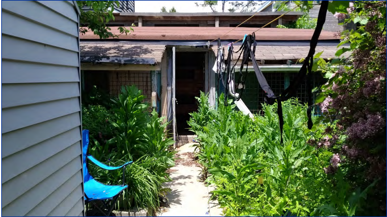
Figure 29: View north of 40 Mitchell Avenue yard shed
