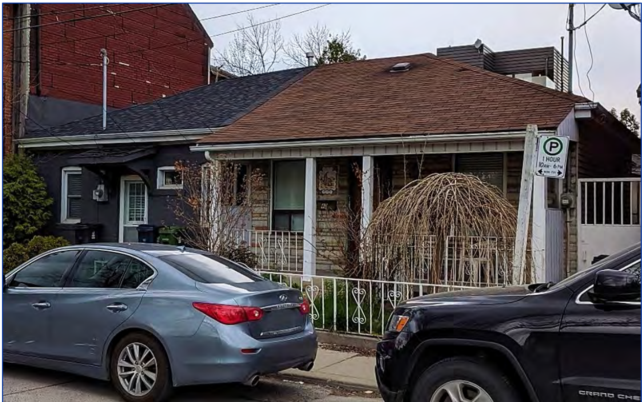
Figure 28: View northeast of façade, 40 Mitchell Avenue on the right
