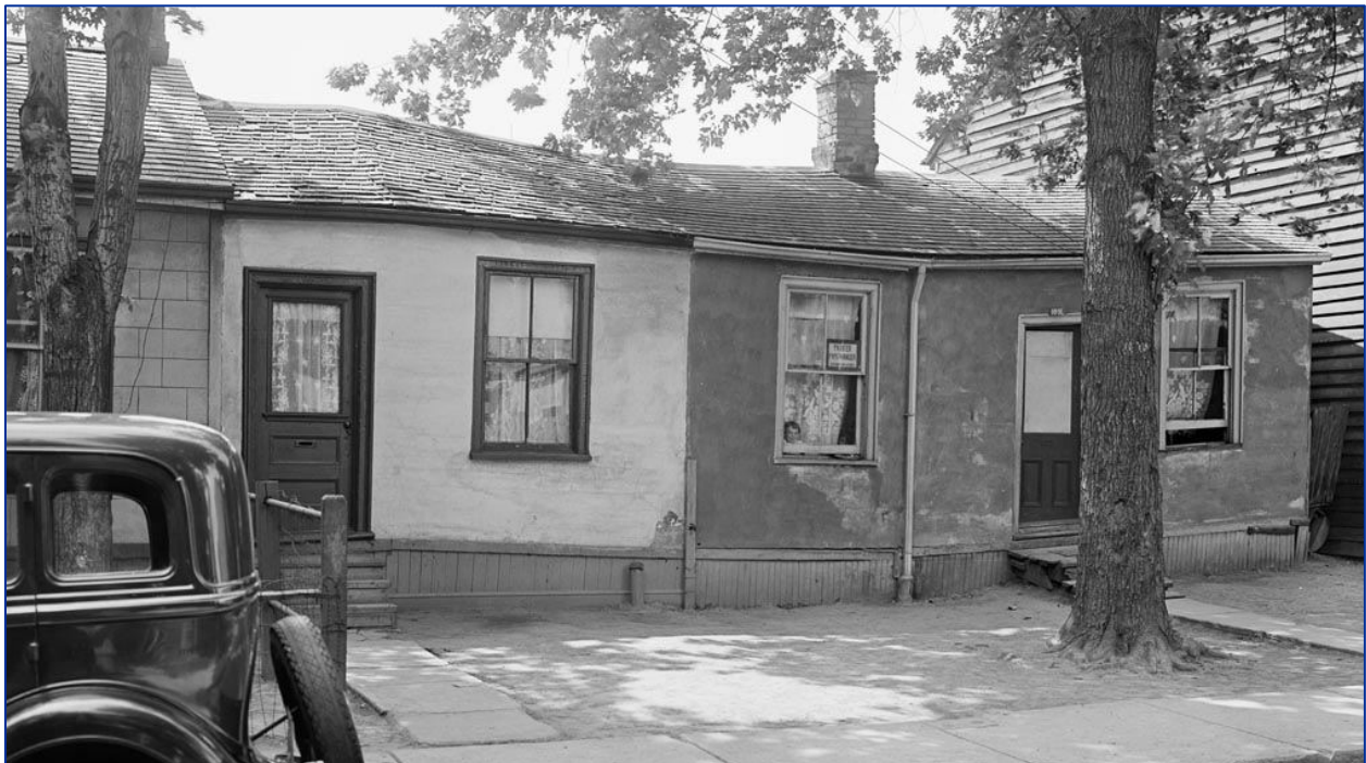
Figure 16: Façade of 63-65 Mitchell Avenue in 1936 61
