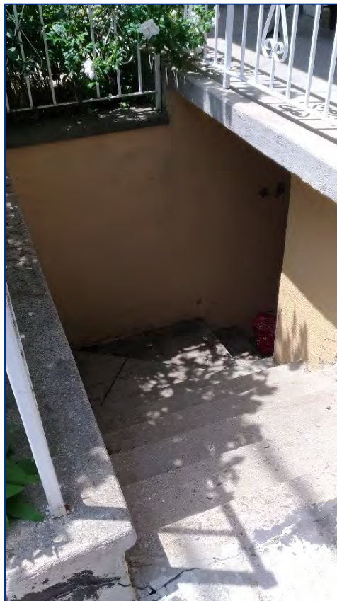
Figure 34: View of stairs down to 40 Mitchell Avenue basement
