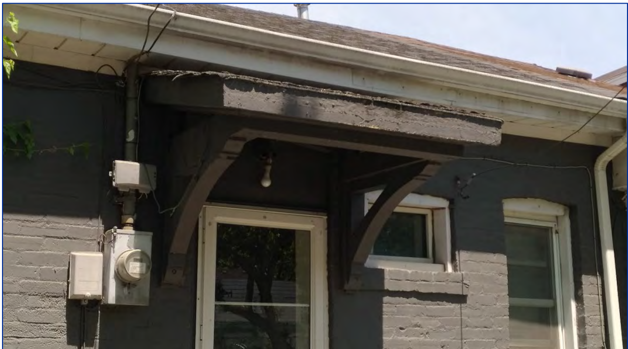
Figure 39: View north of 44 Mitchell Avenue shed style roof
