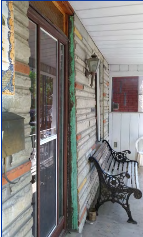
Figure 31: View east of 40 Mitchell Avenue front façade cladding
