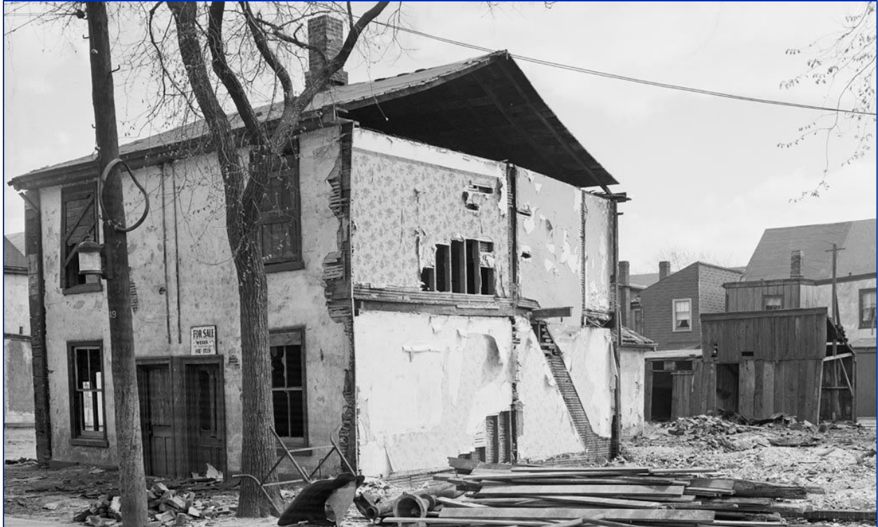
Figure 13: Façade of 43-45 Mitchell Avenue in 1936 58
