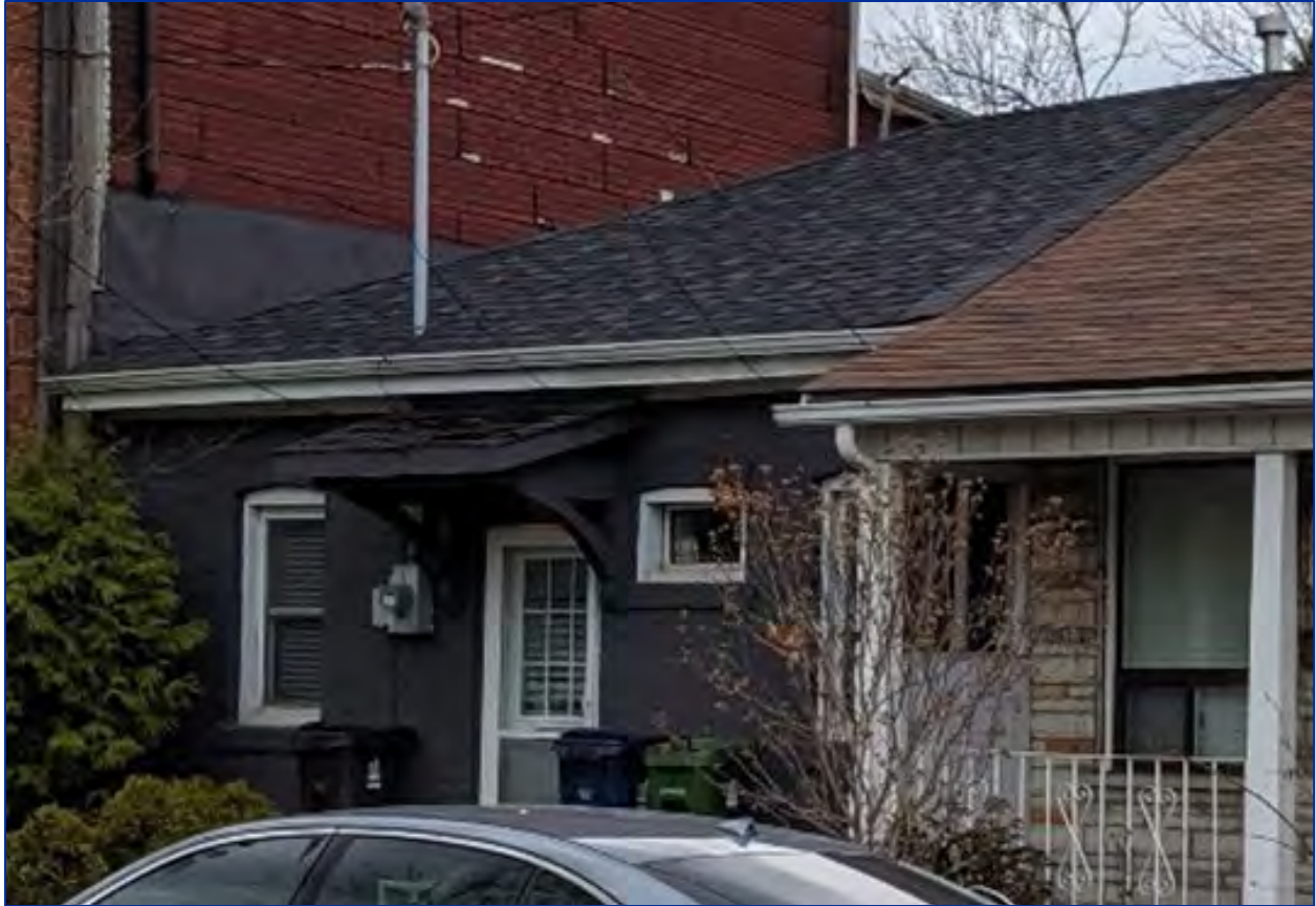
Figure 38: View north of 44 Mitchell Avenue windows and door
