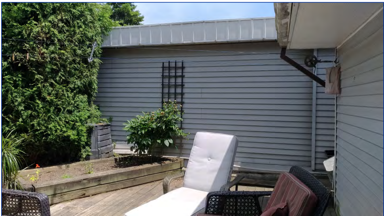
Figure 37: View east of exterior vinyl siding from 44 Mitchell Avenue backyard
