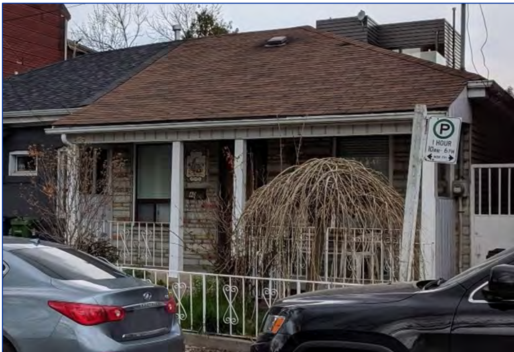
Figure 32: View north of 40 Mitchell Avenue windows and porch
