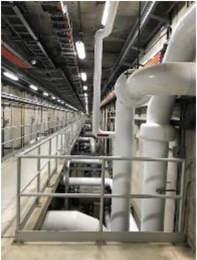
R.L. Clark Water Treatment Plant
