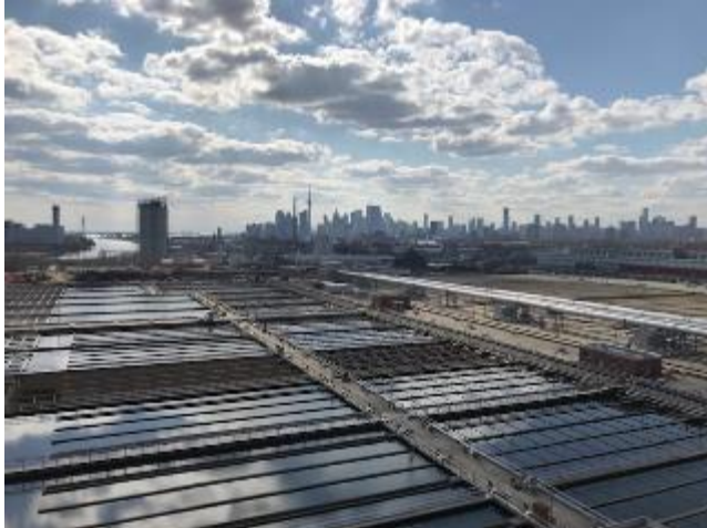
Ashbridges Bay Treatment Plant – aeration tanks
