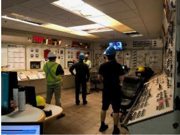
Highland Creek Treatment Plant – control room
