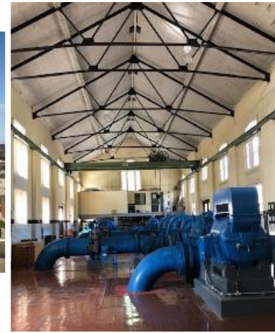
High Level Pumping, Cottingham Street
