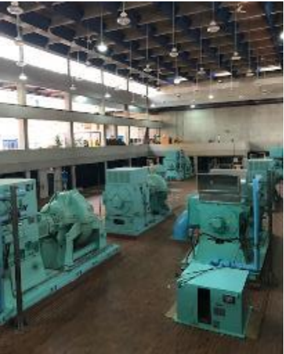
F.J. Horgan Water Treatment Plant
