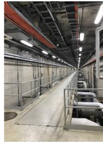
R.L. Clark Water Treatment Plant
