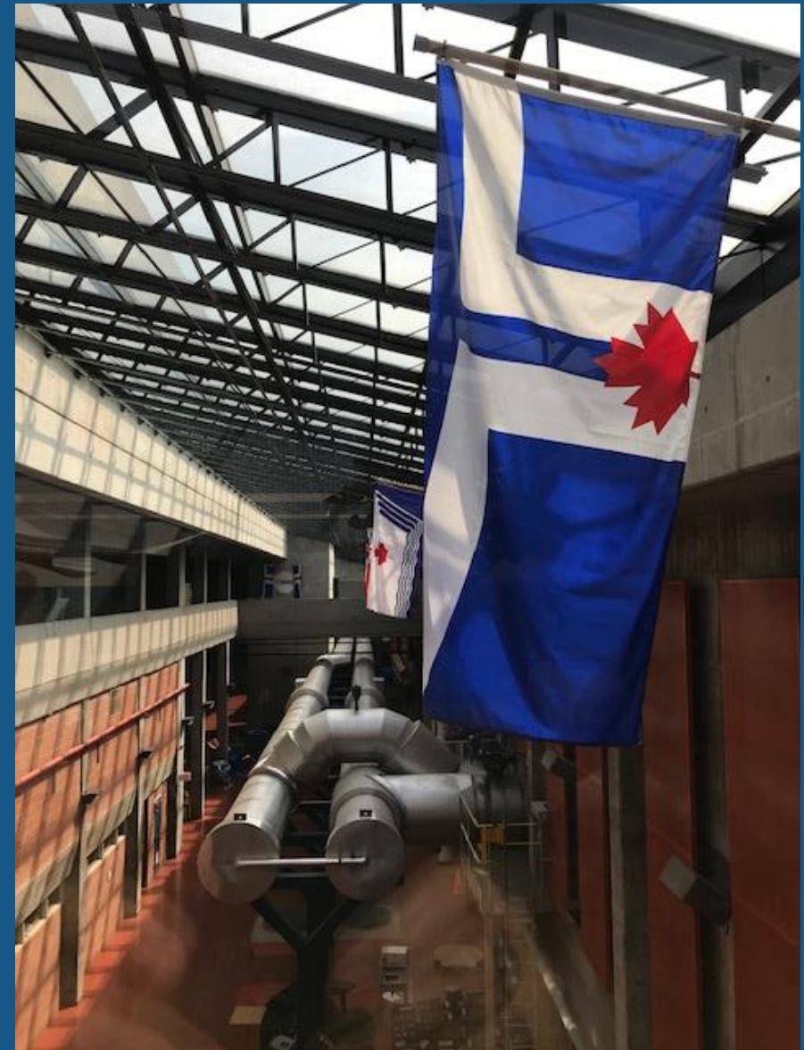
F.J. Horgan Water Treatment Plant
