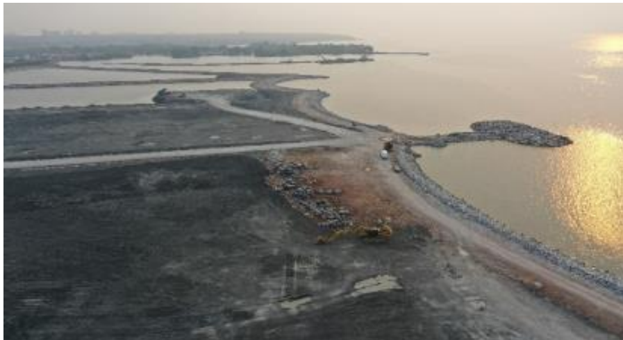
Don River and Central Waterfront & Connected Projects Landform for erosion and sediment control Ashbridges Bay Wastewater Treatment Plant Joint project - Toronto Water & TRCA
