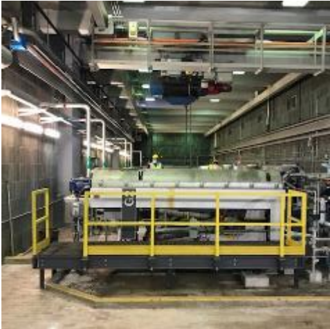
Wastewater treatment plant centrifuges
