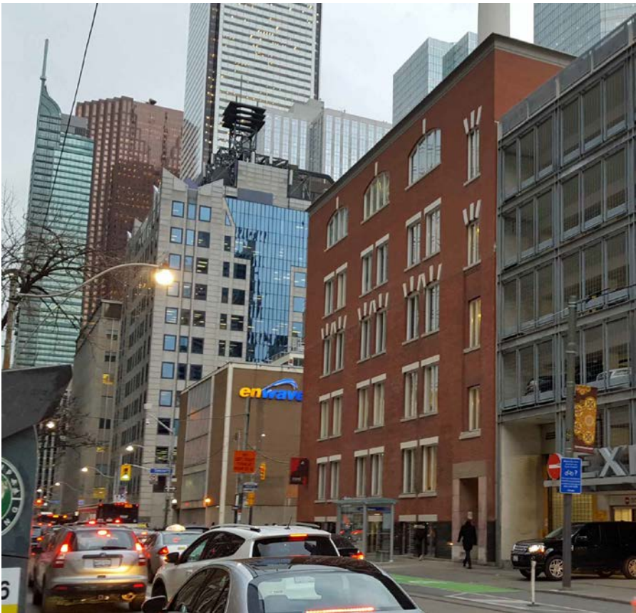
100 Simcoe Street - Adelaide Street West frontage
