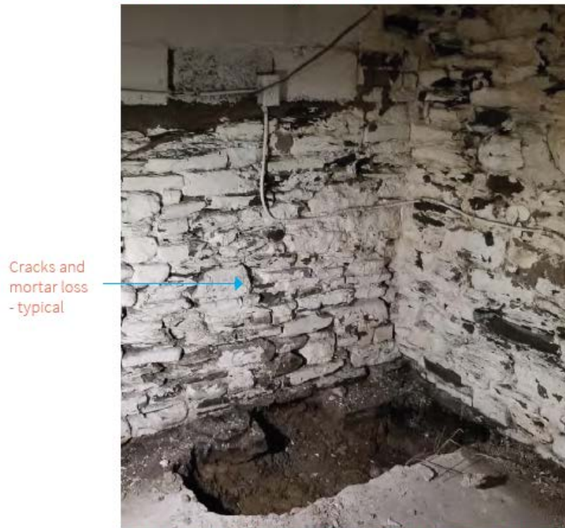
Stacked rubble foundation at 265 Queen Street East - typical (ERA 2018)
