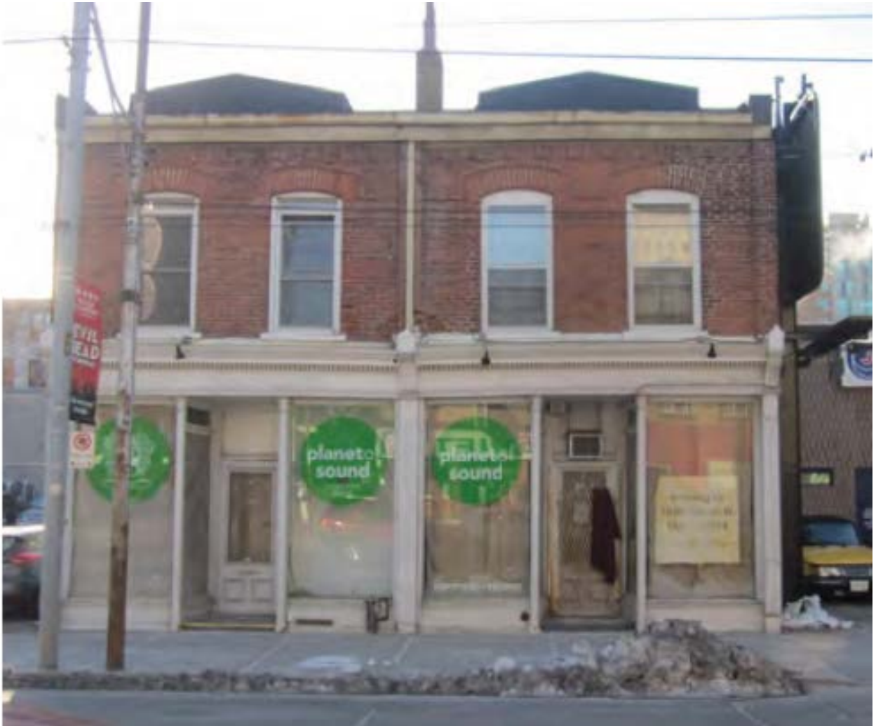
263-265 Queen Street East – existing condition
