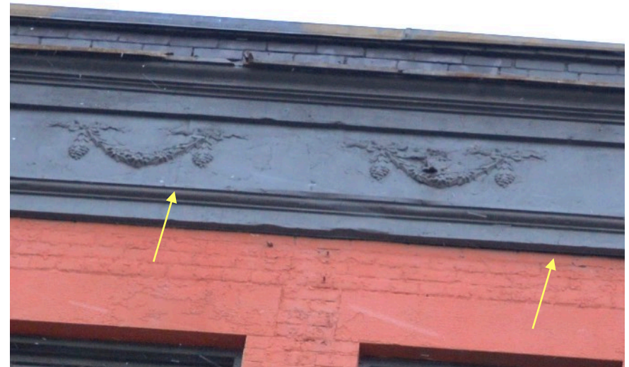
Close-up view of the entablature, showing the decorative festoons. Note the seams of the wooden frieze which vary in their locations. Removal of pieces will need to consider these conditions to avoid damage to festoons located in front of seams. There appears to be plaster or epoxy applied throughout portions of the wooden frieze to mask any potential imperfections of the wood, although the plaster is crudely applied. The metal flashing of the cornice is generally bent and corroded.
