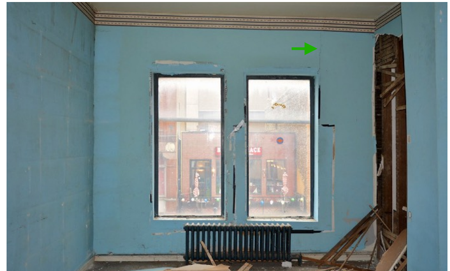
3rd storey interior view. Note the cracking above the window (arrow) and the visible displacement of the wall towards the right (center of the facade).
