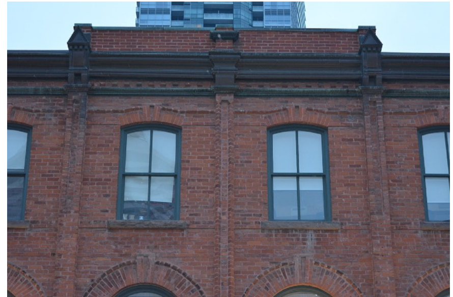
Close-up of the upper storey and the parapet wall. Note the staining due to water runoff under the sills, which themselves are soiled. Soiling is also present at the top of the brick pilasters.
