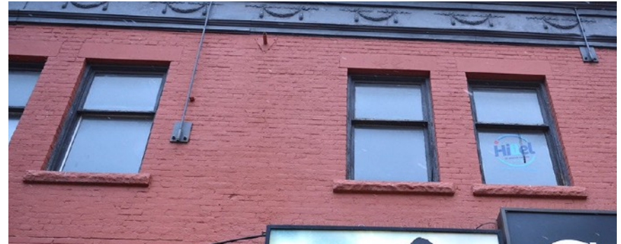
Examples of windows on the Elm Street facade. Windows are of wood, double hung, with the lower sash larger than the upper sash.
