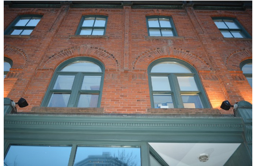
Close-up of the upper storey windows. At the second storey, the windows consist of a pair of double hung windows separated with a thick mullion at the center, and topped with a fixed semi-circular transom. At the third storey, windows are double hung, with a vertical muntin bar on each sash.
