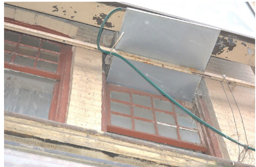
View of second storey windows. The upper sash has been lowered to include what appears to be an air conditioning unit. Note the bird droppings on the glass and the painted wood surfaces.
