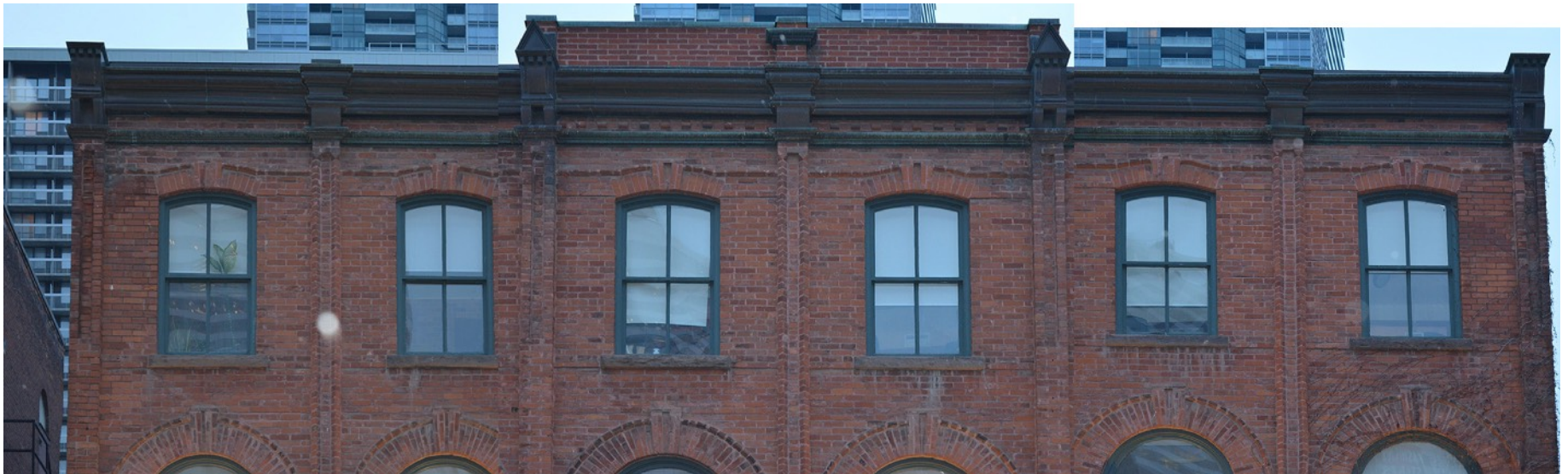
Close-up of the upper cornice and brick parapet (collage photograph)
