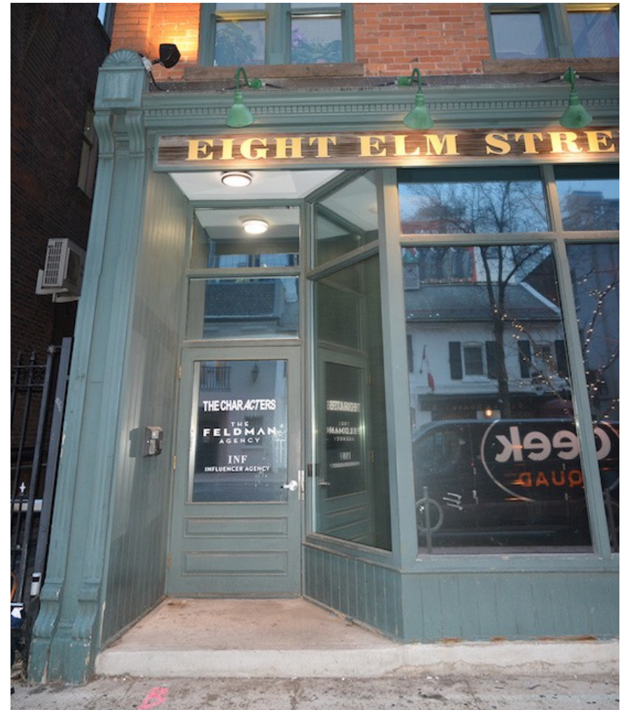
Close-up of the storefront's western entrance. Note the flaking paint near the edges of the bases as they touch the ground as well as at edges overall. These conditions are typical throughout the storefront.
