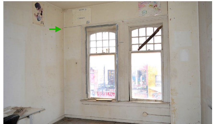
3rd storey interior view. Note the cracking above the window (arrow) and the visible displacement of the wall towards the left (center of the facade), evident by the sloping window sill.
