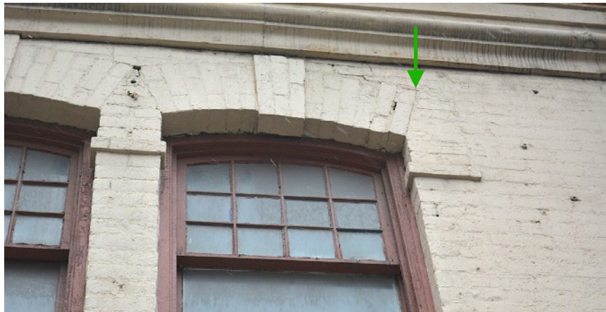
View of a second storey window showing the visible displacement of the lintel (green arrow). Stepped cracking is also notable above the lintel. Note the many holes on the facade, previous locations of anchors to secure signage.
