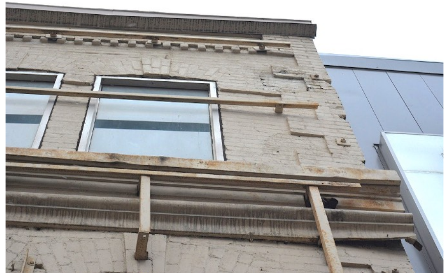
Close-up views of pressed metal cornice between the second and third storeys, which is punctured in some locations for signage structure. The cornice is bent, dirty and corroded at the top.
