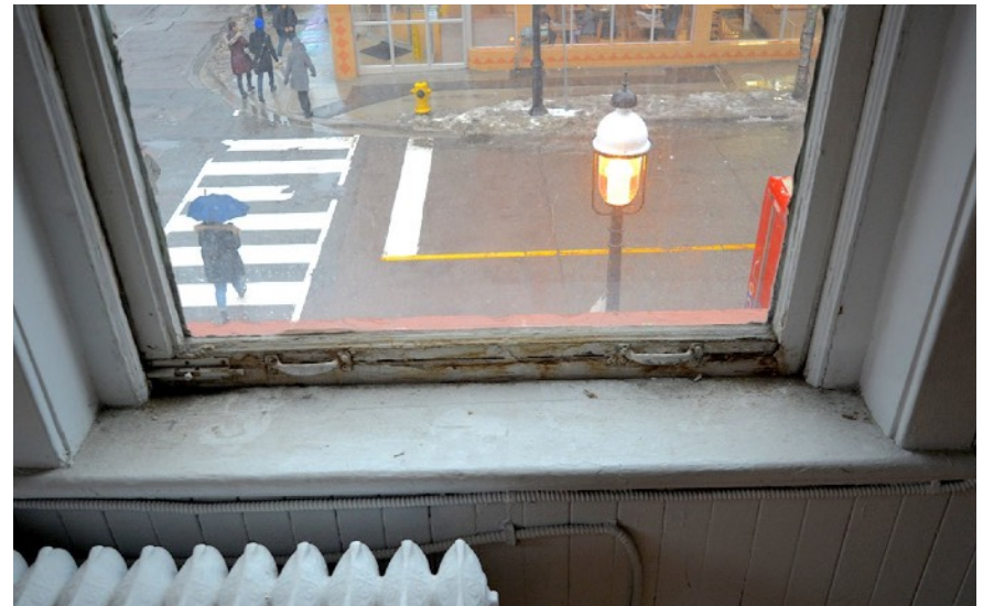
Example of a lower sash with its bottom rail heavily deteriorated.
