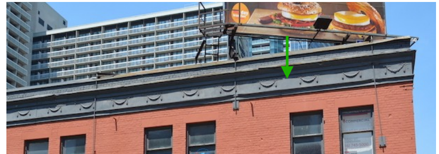
Overall view of the entablature along Elm Street. Note the metal anchors that have damaged the metal cornice and architrave moulding
