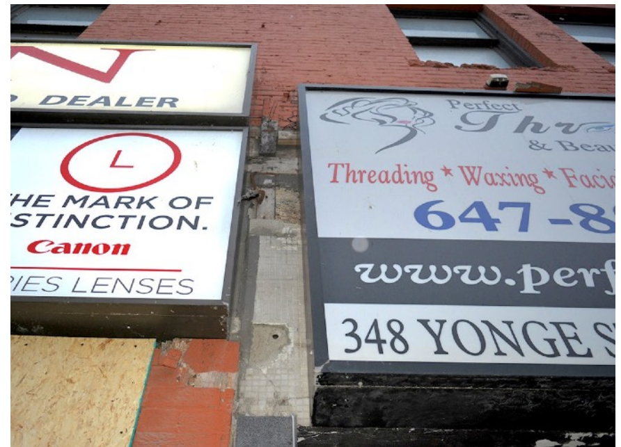
Close-up view of the condition between signage bands, showing a mix of materials resulting from successive alterations. At this location was noted a wooden beam, which appear to be original yet was not fully assessed due to obstructions of the signage bands.
