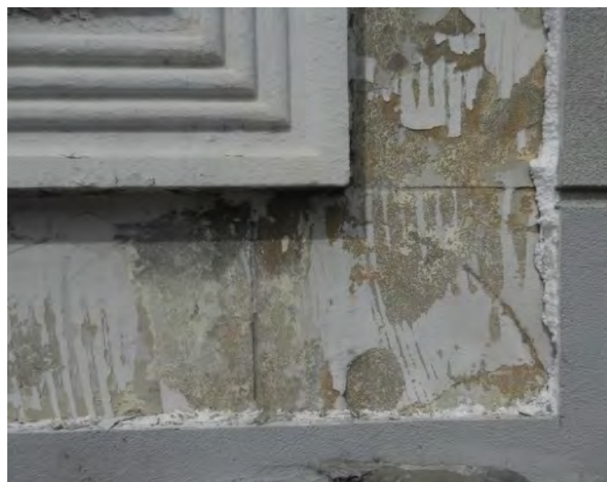
Opening below the window frame on the second level. The stucco/ expanded polystyrene was applied over what appeared to be stone panels (joints/seams are noticeable). Further removal of the bonding agent will be removed as part of the conservation treatment, by scraping and further by cleaning.
