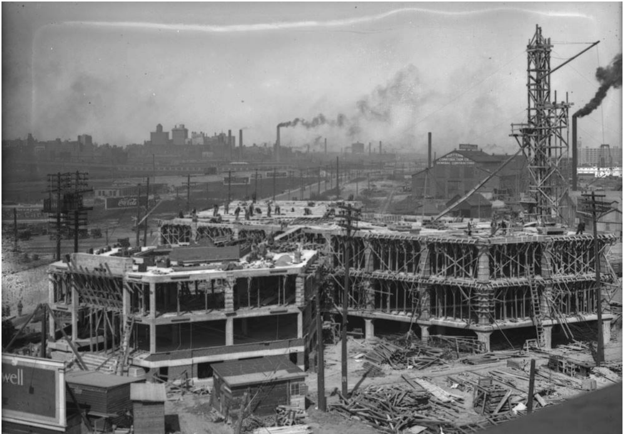
Figure 16: The subject property under construction, 1927. (Toronto Harbour Commissioners / Library and Archives Canada / PA-098619 – MIKAN 3656094 – 1927.)
