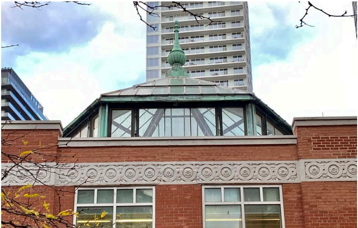
Figure 42: 545 Lake Shore Boulevard West; details of the glazed lantern atop the hexagonal pavilion and decorative cast-stone banding. (Heritage Planning, 2021.)
