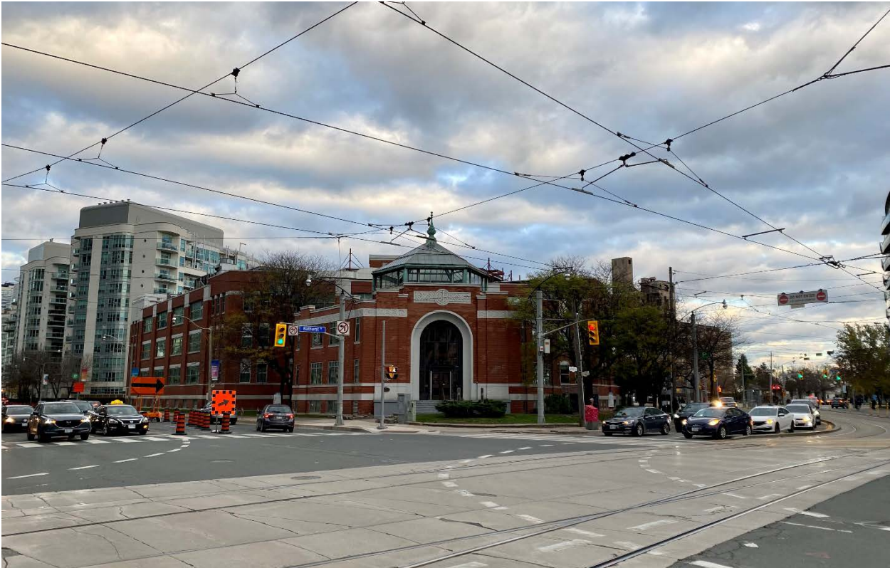
Figure 1: 545 Lake Shore Boulevard West; view of the property's northwest corner from the intersection of Lake Shore Boulevard West and Bathurst Street. (Heritage Planning, 2021.)
