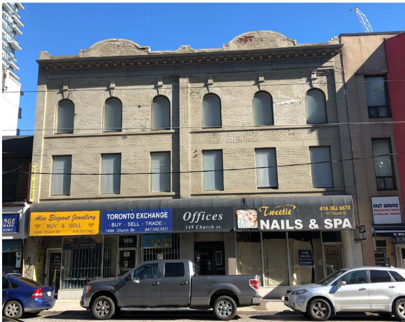
West (principal) elevation of 147 Church Street (Heritage Planning, 2021)
