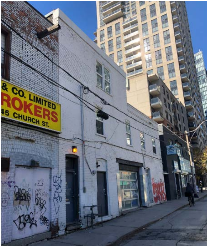
15. Current photograph looking northwest on Dalhousie Street, showing the rear (east) elevation of the building at 147 Church Street (this elevation contains the entrance addresses at 18 and 20 Dalhousie Street). (Heritage Planning, 2021)
