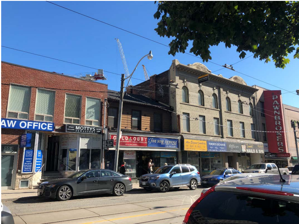
14. Current photograph looking southeast on Church Street, showing the principal (west) and side (north) elevations of the building at 147 Church Street. (Heritage Planning, 2021)
