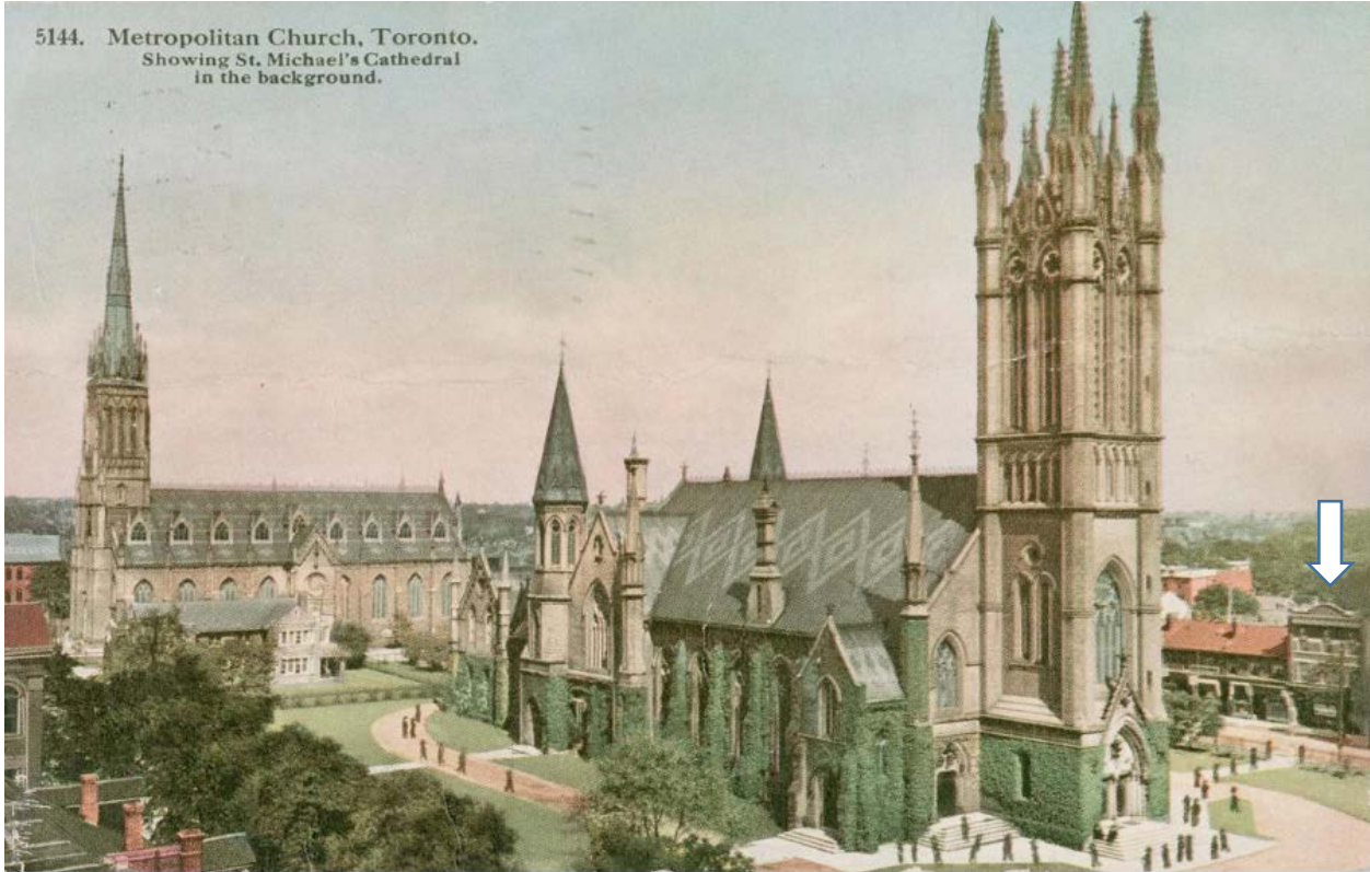
9. 1914 archival photograph of the Metropolitan Church and St. Michael's Cathedral, with the existing three-storey mixed-use/commercial property at 147 Church Street shown on the far right of the image. (TPL)
