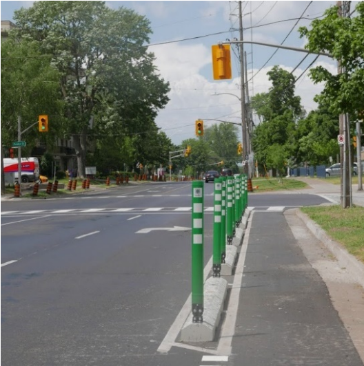
Flexible Bollards Mounted on Pre-Cast Concrete Curbs
