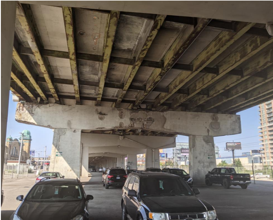
Under the Gardiner at Parking Lots and Storage Areas
