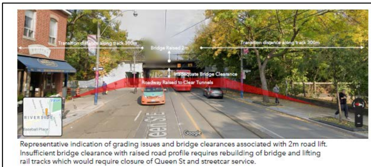
Figure 4. Options 1 and 4 - 4.5% Grading Road and Bridge Clearance Impact (Source: Metrolinx/Infrastructure Ontario).
