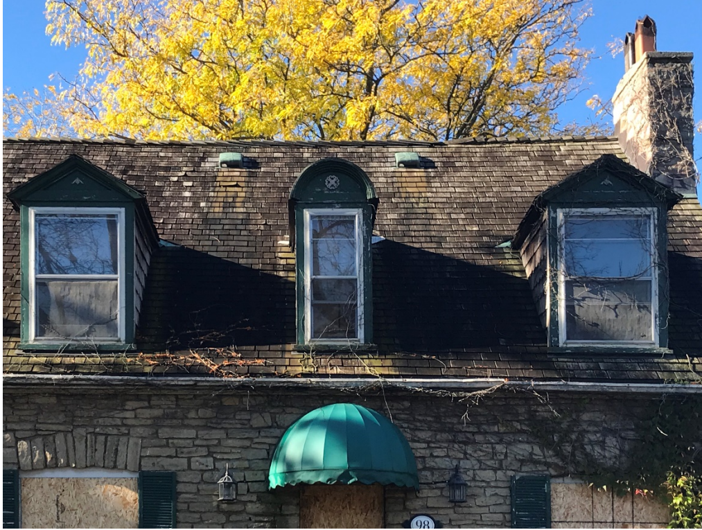
8. Current photograph of 98 Superior Avenue showing the neo-classically inspired dormer window roofs. Note: at the time of writing this report, the property has been boarded up. (Heritage Planning, 2020)
