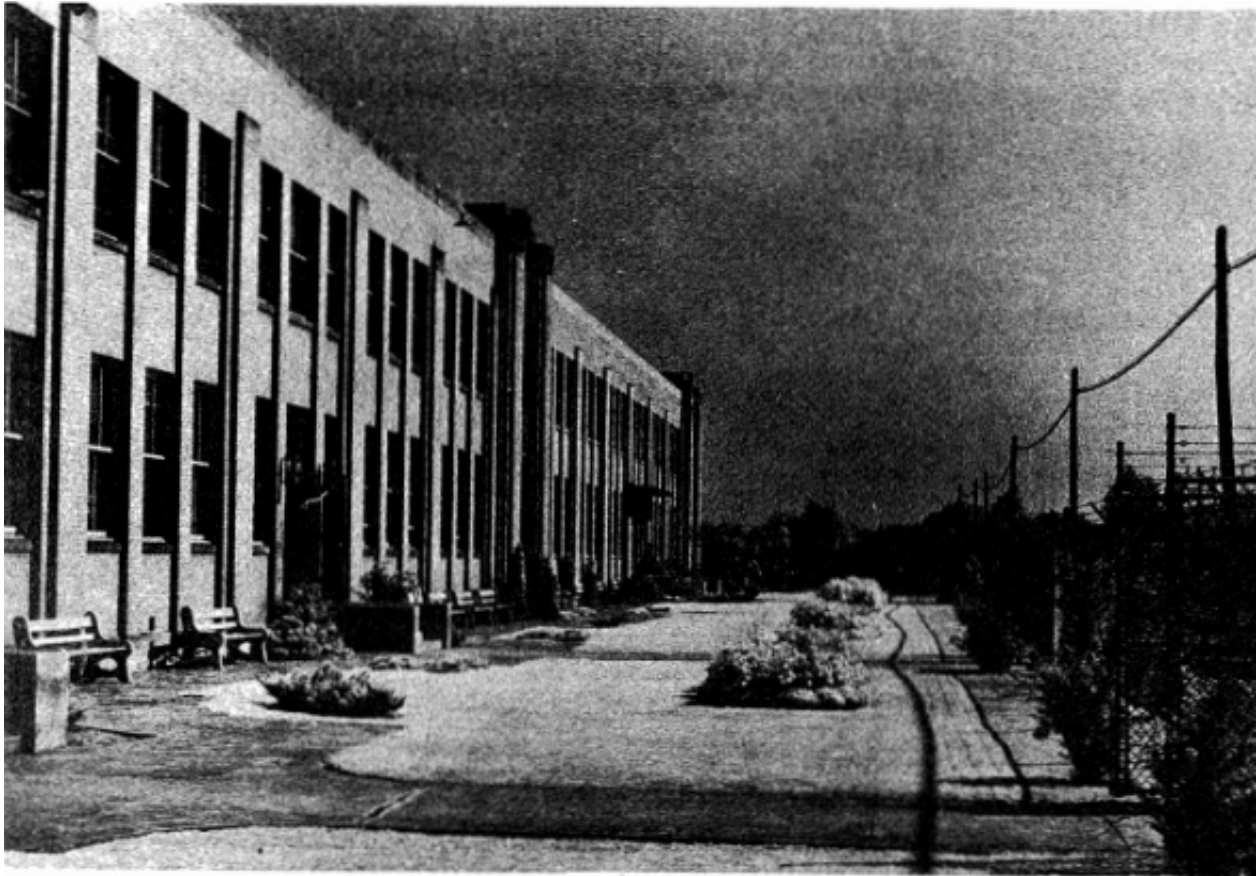
Figure 13. Image of the principal (south) elevation of the 1931 and 1944 manufacturing building (1951) (Courtesy of the City of Toronto Archives)
