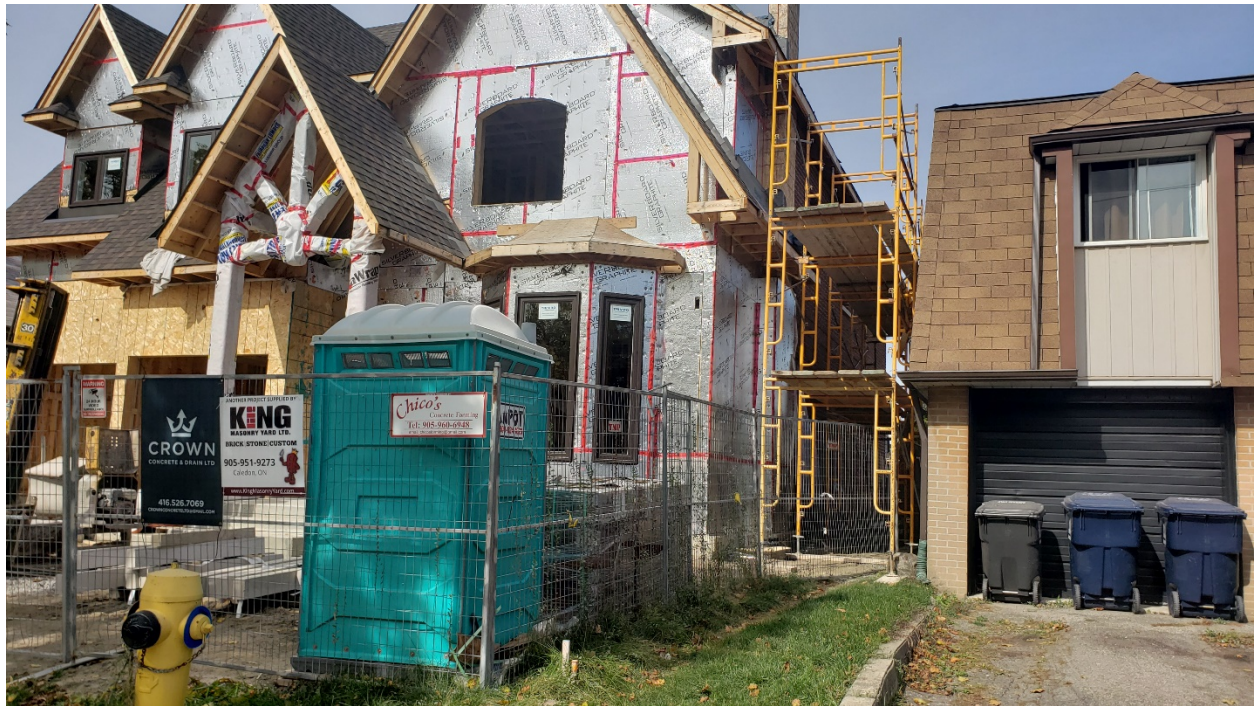
Attachment #1-Front facing, fence to be where scaffolding is located, east side
