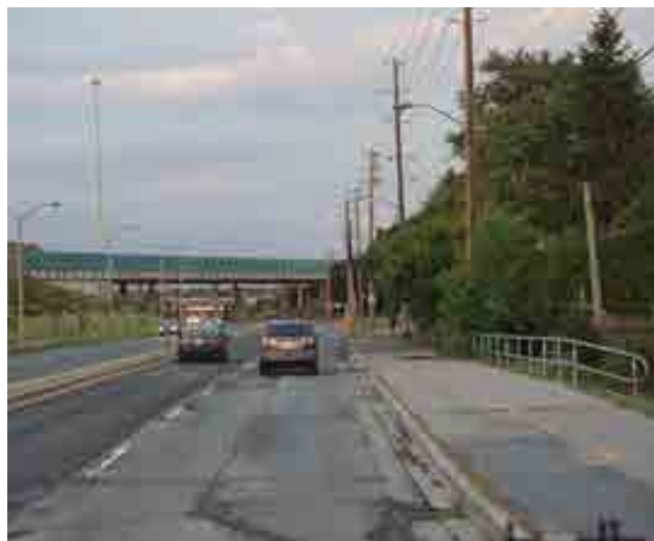
Figure 36. Close Proximity/Lack of barrier between existing multi use path and vehicular roadway
