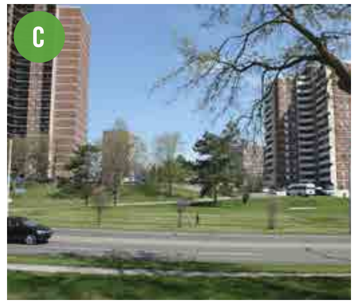
Figure 51. View of apartment buildings on the north side of Eglinton Avenue
