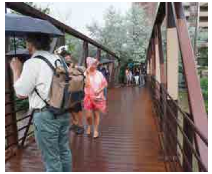
Figure 27. Pedestrian bridge east of future location of Mulham Station
