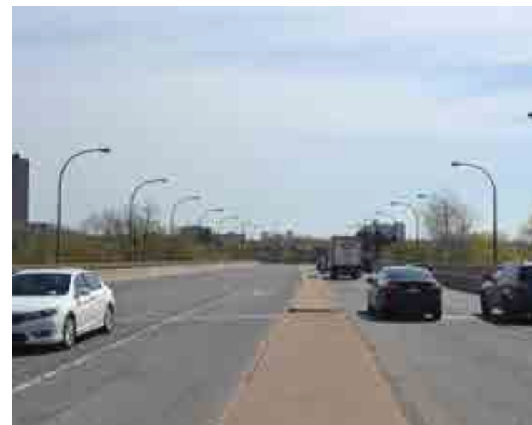
Figure 38. Center roadway in some sections along Eglinton Avenue
