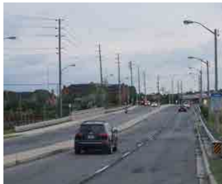
Figure 37. Roadway travels over channelized Mimico Creek
