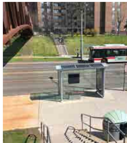
Figure 22. Bus shelter on Eglinton Avenue
