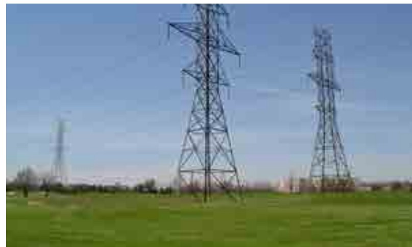
Figure 125. Hydro corridor adjacent to Martin Grove Road
