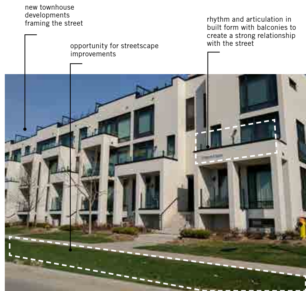
Figure 132. New townhouse development on Widdicombe Hill Boulevard
