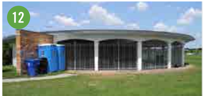
Figure 92. Richview Pumping Station
