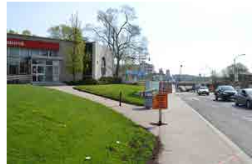
Figure 172. Some areas have manicured landscaping
