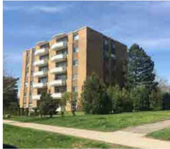
Figure 69. Six-storey multi-unit housing
