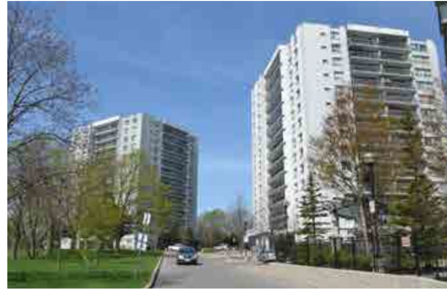
Figure 70. Fontenay Court apartments
