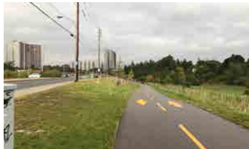
Figure 126. Multi use path on south side of Eglinton Avenue West
