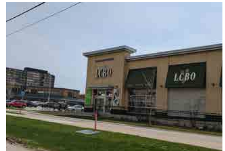
Figure 114. Lloyd Manor Plaza
