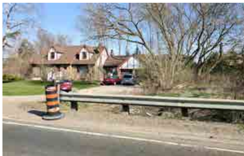
Figure 143. Missing sidewalks along the north of Eglinton Avenue West
