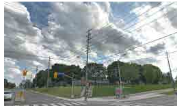
Figure 215. Existing hydro lines crossing intersection of Eglinton Avenue and Islington Avenue
