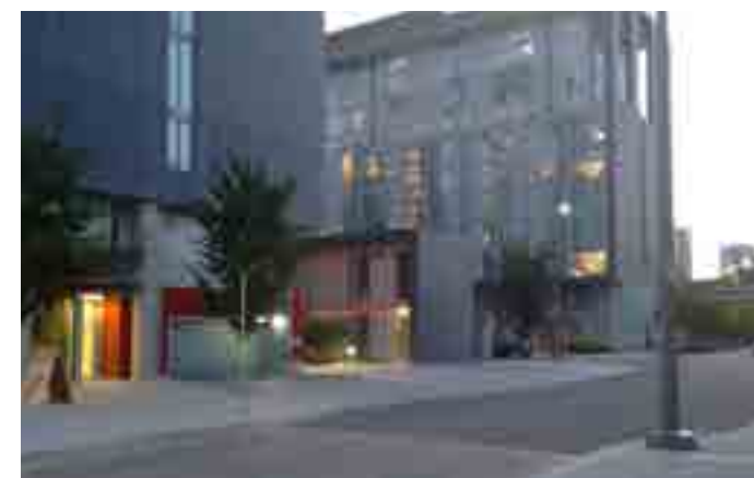
Figure 181. Shared access for pedestrians, cars, and loading vehicles (Athletes' Village, Toronto)
