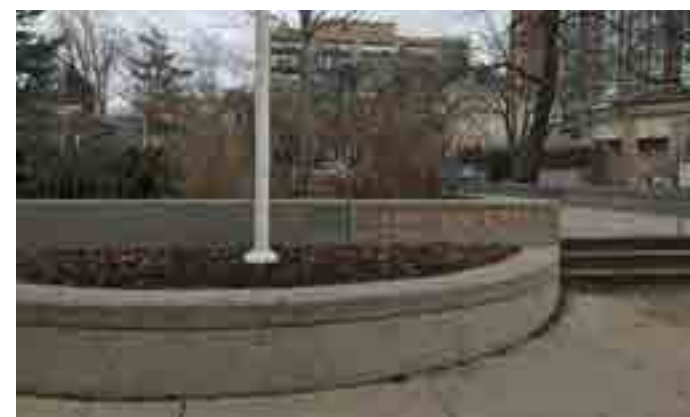
Figure 213. Concrete planters with signage to signify connection to natural features (Wellington Street, Toronto)
