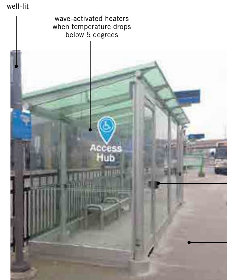
Figure 190. The TTC's first Access Hub at the Meadowvale loop is the first of 12 hubs across the city. Note: shelters along Eglinton West will have side doors rather than front doors.
