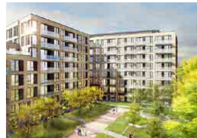
Figure 240. Mid-rise residential with outdoor amenity space, Montreal
