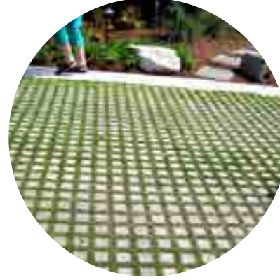
Figure 224. Pervious grid pavement solution for driveways and mid block connections
