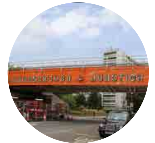
Figure 204. New painted bridge as part of a project to celebrate local identity (Loughborough, London)
