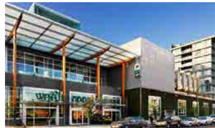
Figure 241. Mixed-use development (Vancouver)
