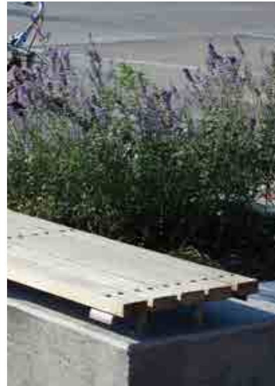
Figure 263. Seating integrated in planters, Greensburg Main Street, Kansas City, MO (image credit BNIM)
