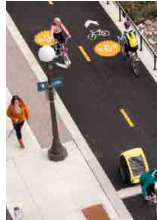
Figure 264. Buffer between pedestrians and cyclists, Jackson Street, Saint Paul (image credit Toole Design)
