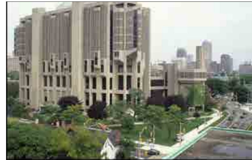
Figure 358. Roberts Library designed in 1973 by Warner, Burns, Toan and Lunde and Mathers and Haldenby (City of Toronto Archives, Fonds 200, Series 146, File 212, Item 2).
