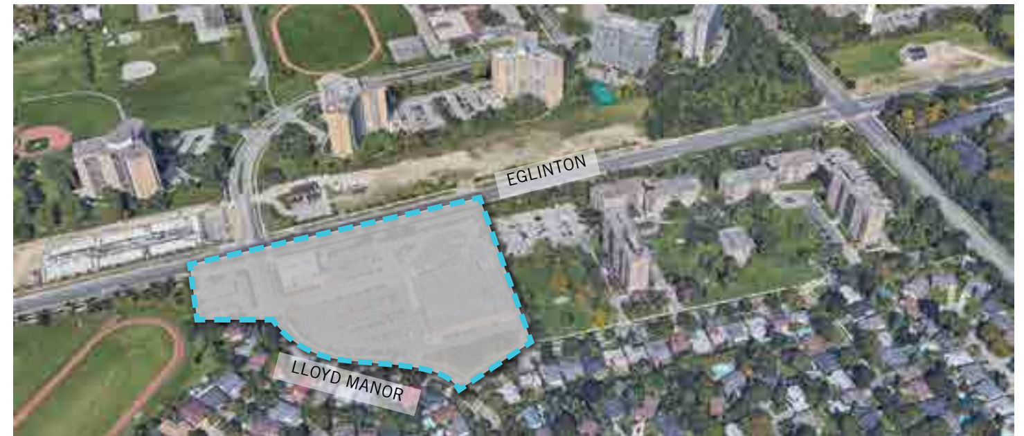
Figure 403. Bird's eye view of Lloyd Manor Plaza Site
