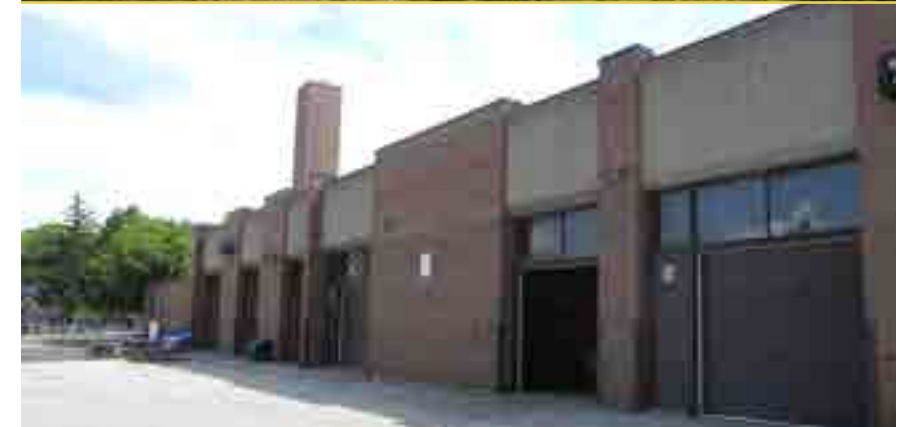
Figure 363. Richview Pumping Station and Central Etobicoke High School (Common Bond Collective, August 2018).
