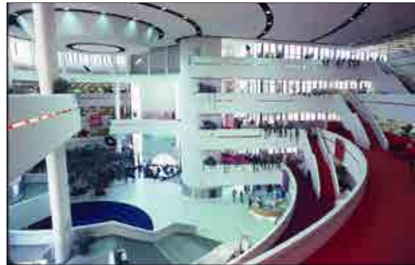
Figure 357. Interior of Scarborough Civic Centre designed by Raymond Moriyama in 1973 (City of Toronto Archives, Fonds 200, Series 1465, File 97, Item 14).
