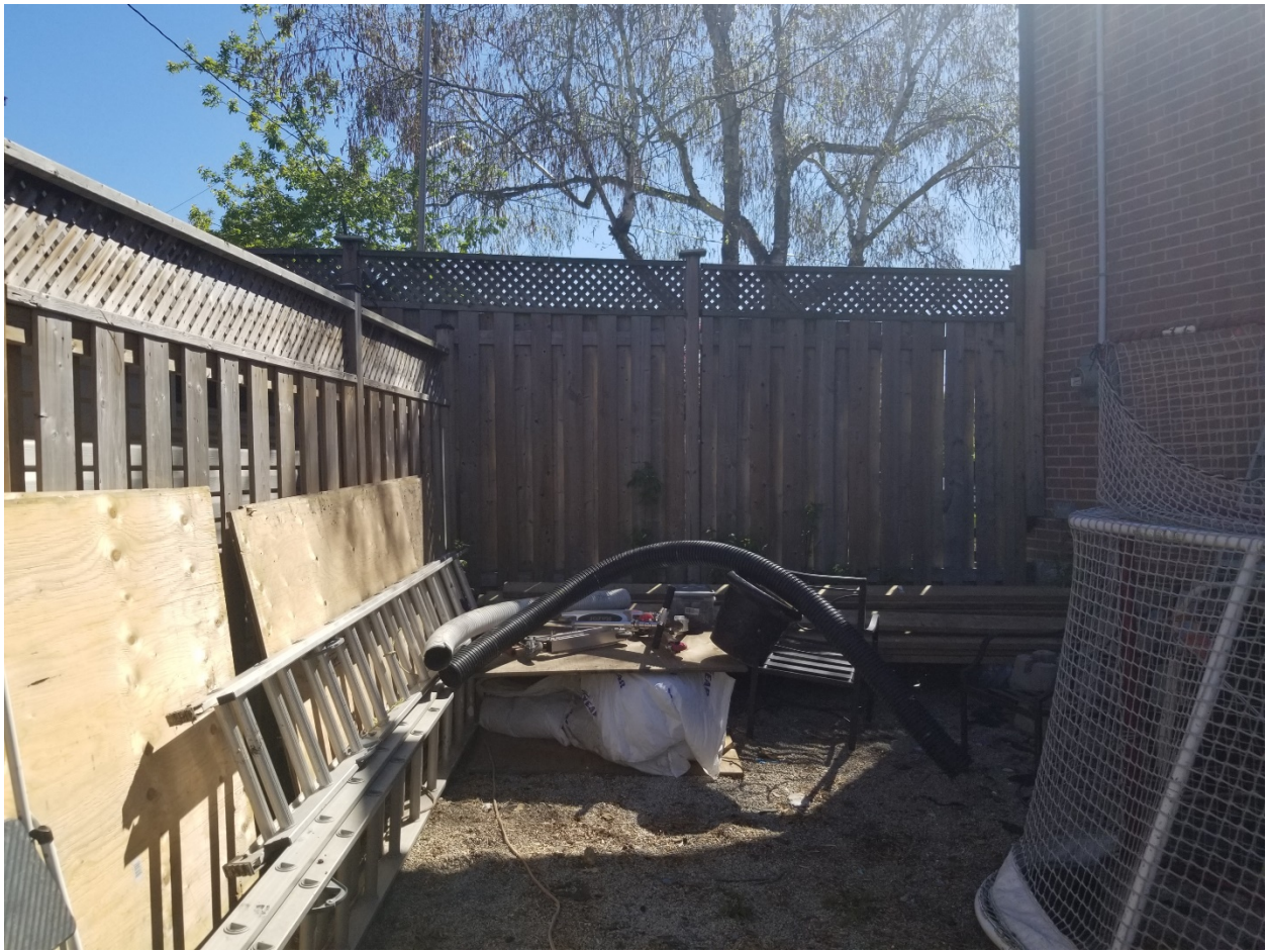
Attachment 2: East Fence (photo taken facing East)
