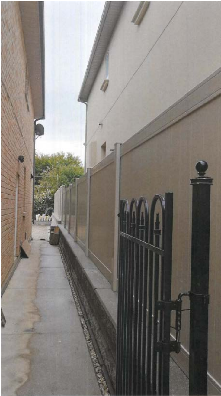
Attachment 3: PVC fence on West side of property (photo taken facing South)
