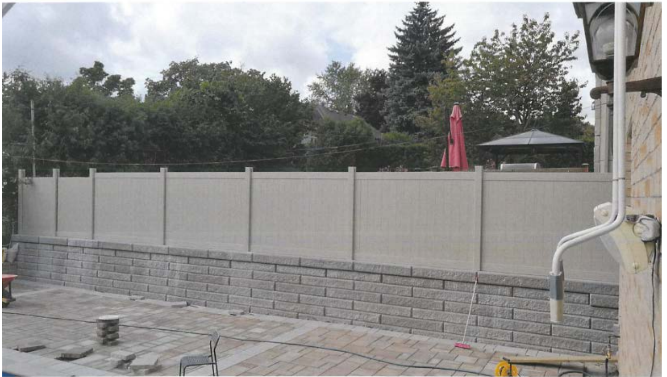
Attachment 2: PVC fence installed on West side of property (photo taken facing South-west)
