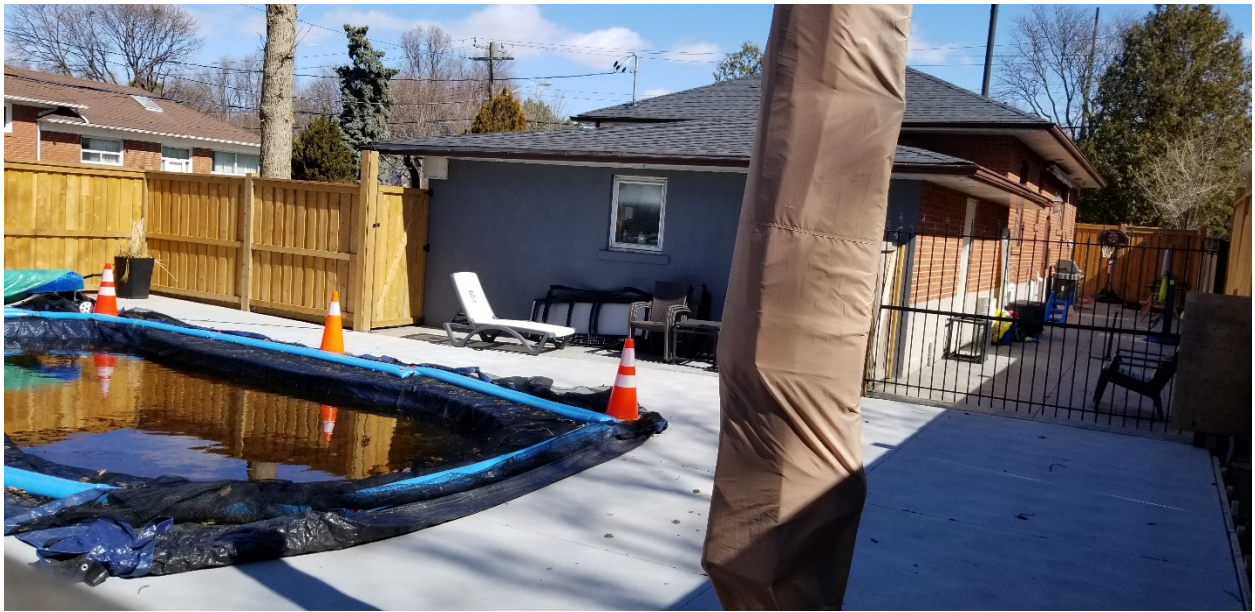
Attachment 5: Swimming pool enclosure using the garage as part of the enclosure (photo taken facing east)
