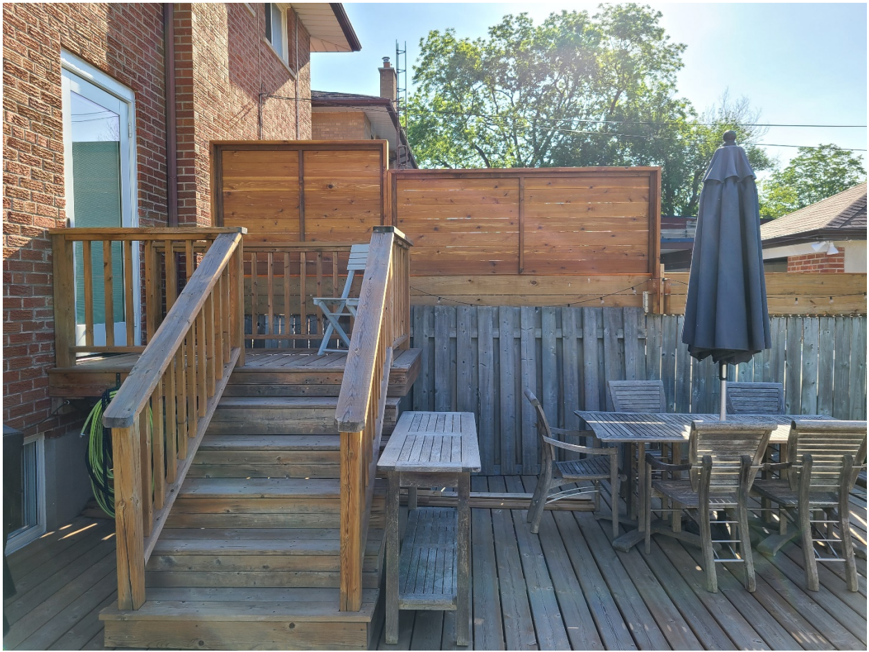
Attachment 2: Rear Fence (photo taken facing East)
