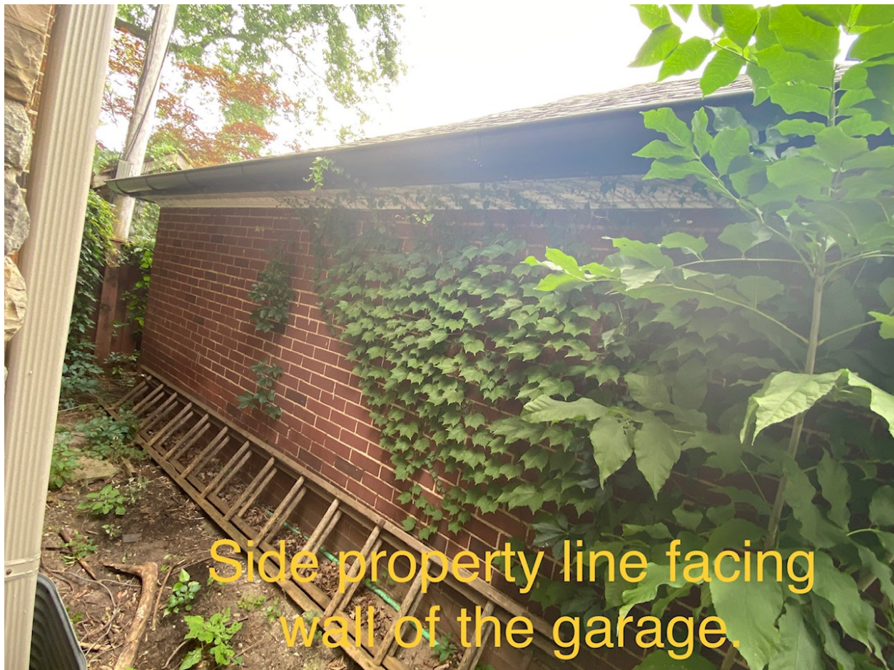
Attachment 4: Photograph submitted by applicant indicating side property line
