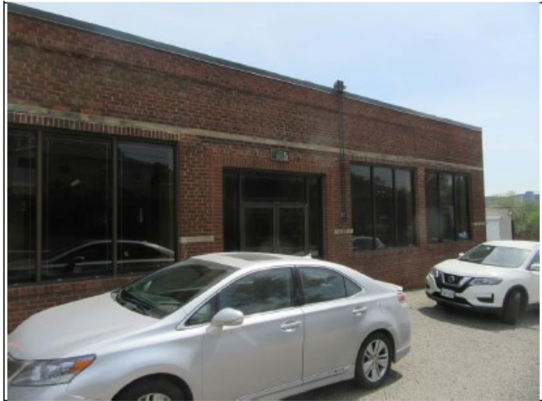
PHOTO NUMBER 1: Front view of 975 Weston Road
