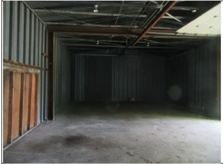
PHOTO NUMBER 5: Interior view of steel shed
