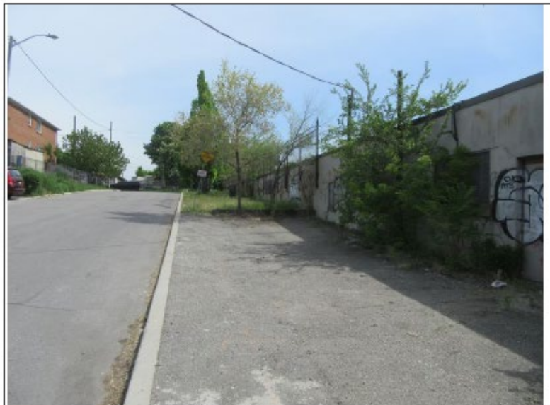
PHOTO NUMBER 6: North exterior wall and adjacent street sloping up.
