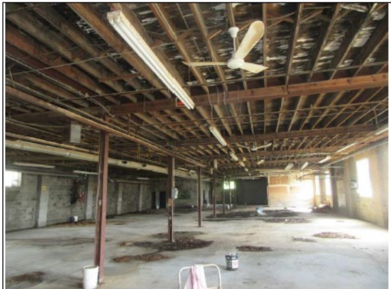
PHOTO NUMBER 2: Interior view of structure.
