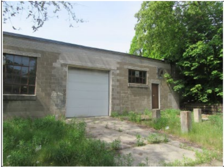
PHOTO NUMBER 3: Rear (east face) of building
