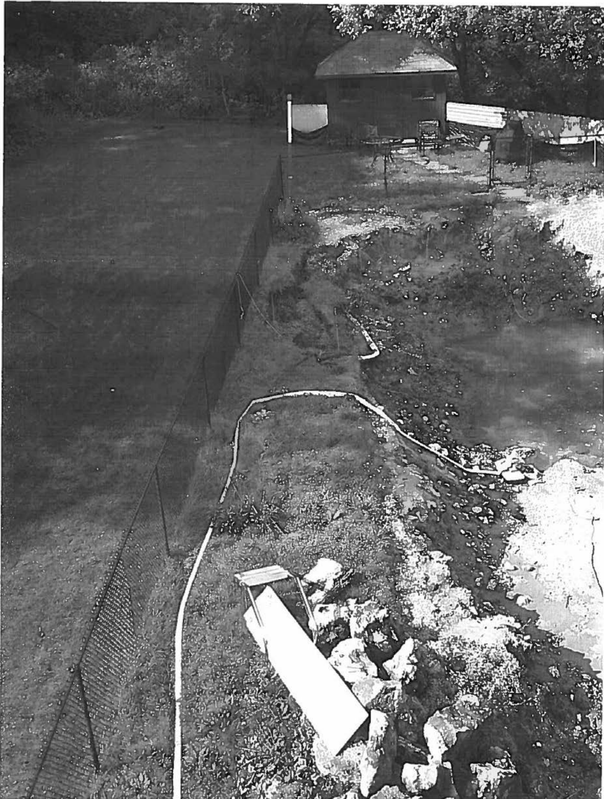
Attachment 3: Rear Yard (photo taken facing North)
