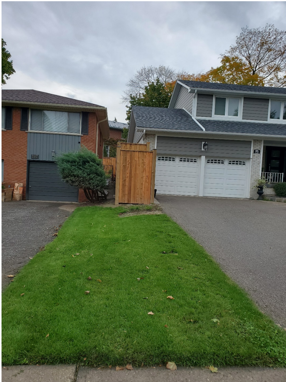
Attachment 2: Front yard fence (facing East)
