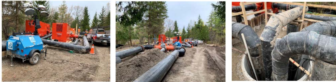
Figure 2: Large scale sewer bypass system
