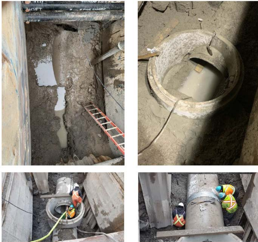
Figure 3: Excavation and repair of the 15 metre STS
