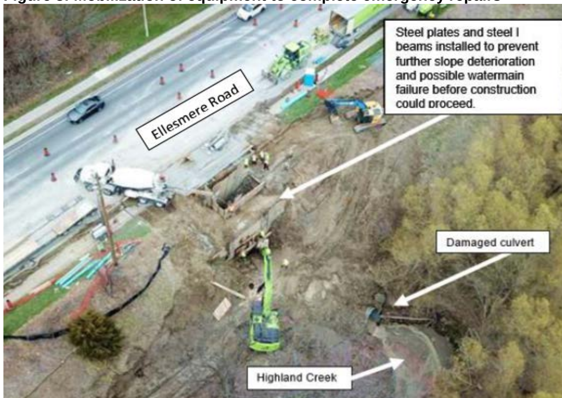
Figure 3: Mobilization of equipment to complete emergency repairs
