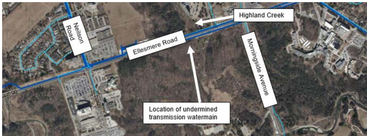
Figure 1: Location of undermined 2100mm transmission watermain
